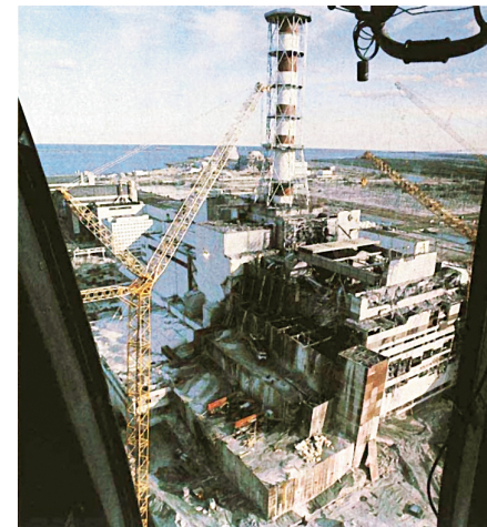
Fig. 2.10.3 The Chernobyl nuclear power plant
