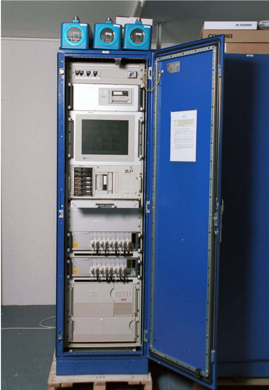
FIG. 30. Digital multi-camera optical surveillance (DMOS) system.
