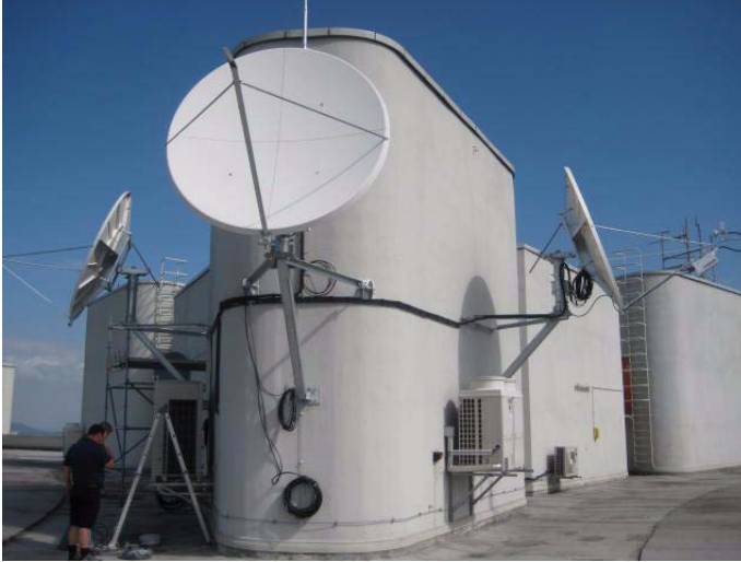
FIG. 43. Satellite antenna at IAEA Headquarters.
