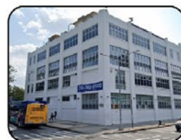
Warehouse and Offices at Tompkins Ave & Flushing Ave.
