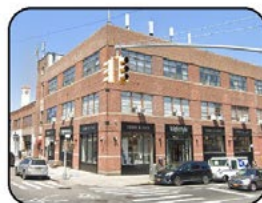
Warehouse and Groundfloor retail at Park Ave. & Franklin Ave.
