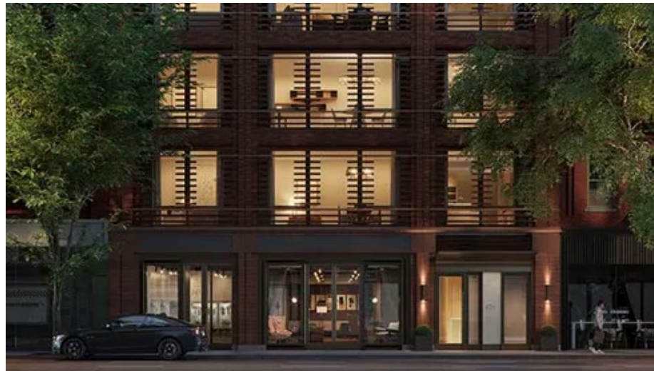
Passive house development
