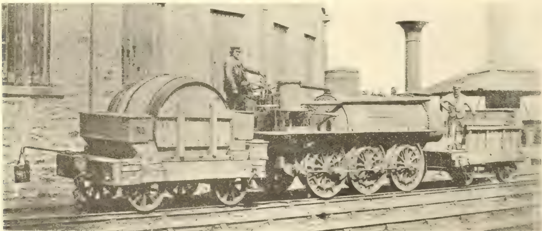
FIG. 21—"WILBERFORCE," STOCKTON AND DARLINGTON RAILWAY, 1831
