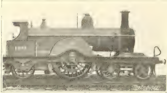
FIG. 330—S. W. JOHNSON'S SINGLE EXPRESS ENGINE, MIDLAND RLY., 1889-93
