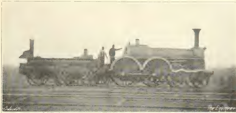
FIG. 138—G.W.R. BROAD GAUGE LOCOMOTIVE "CŒUR DE LION," BY D. GOOCH, BUILT BY R. STEPHENSON & CO., 1855 (From a photo lent by Mr. H. V. Pegg)
