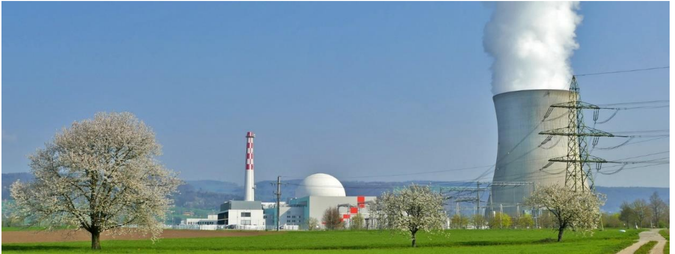
Figure 24.2. Nuclear power plant in Switzerland (Image by ramboldheiner from Pixabay)
