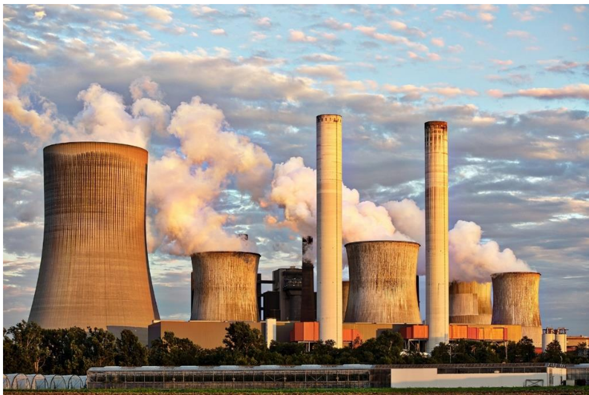
Figure 4.12. Coal fired power plant (Image by Benita Welter from Pixabay)
