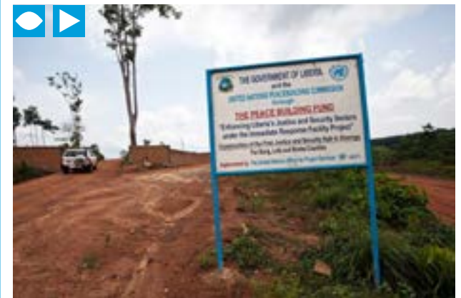
In Gbarnga, construction is underway for a new $3.7 million justice and peace hub, paid for by the UN Peacebuilding Fund and being built by the United Nations Office for Project Services. The facilities will include courts, offices, barracks and training centres for security agencies, and serves much of central Liberia. A sign at the entrance of the Gbarnga Justice and Peace Hub. 13 APRIL 2012/UN PHOTO/STATON WINTER
