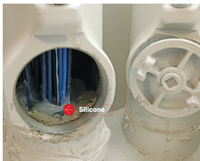
FIGURE 1. Caulking around Service Intrusion*
