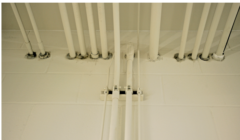
FIGURE 18. Caulking around Service Intrusions*
