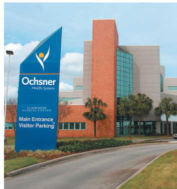
Ochsner Hospital – Elmwood Jefferson, LA
