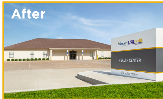
After: Community Health Center, St. Vincent exterior
