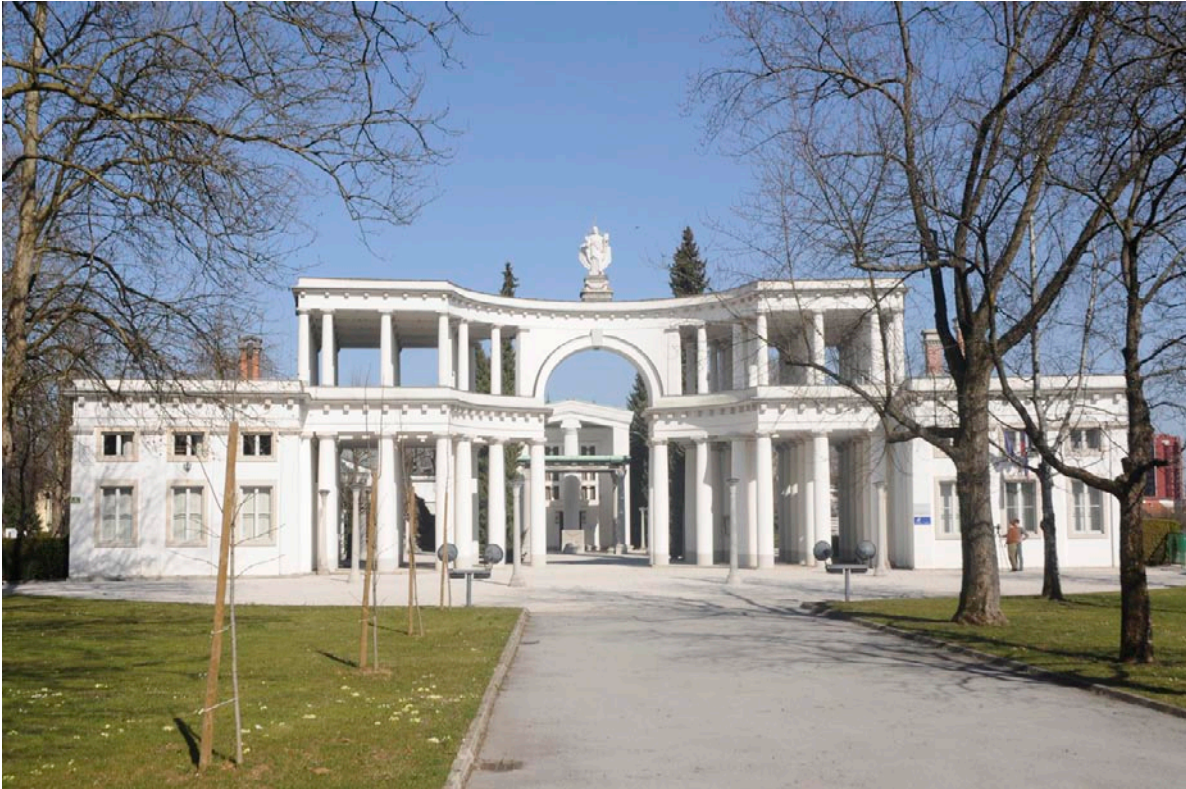
The architect's name is Joze Plecnik and the name of the building complex is Plecnikove Zale (in English Plecnik's Zale).
