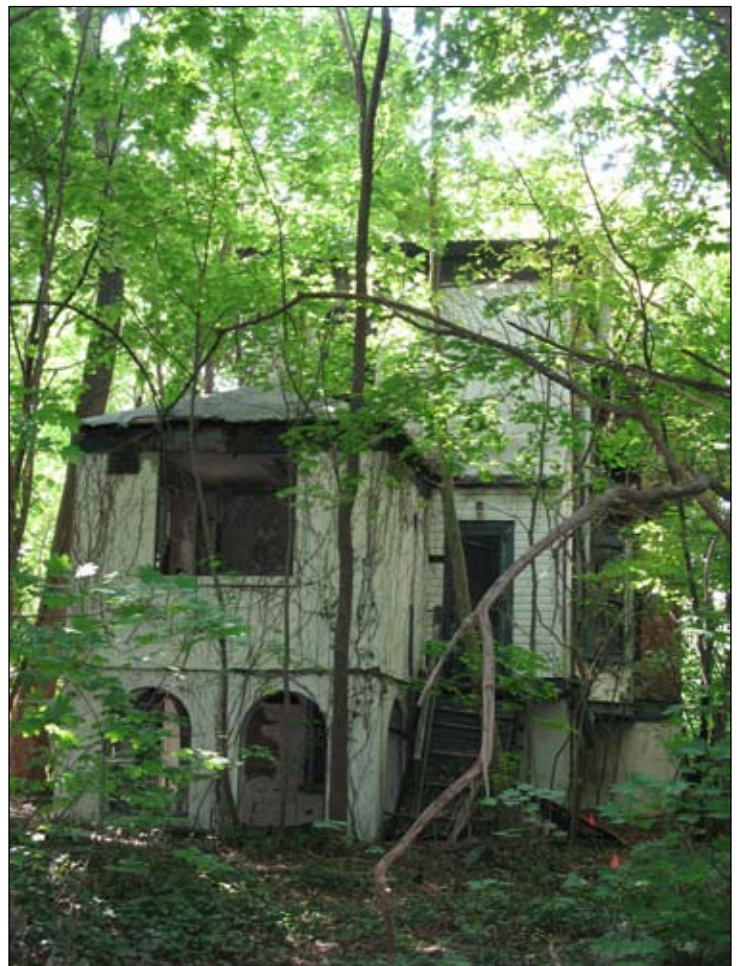
Rear (north) façade 12
