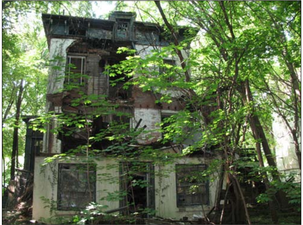
Rear (north) façade 5
