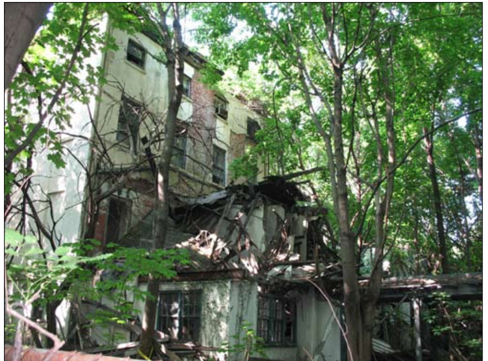
Rear (north) façade 2
