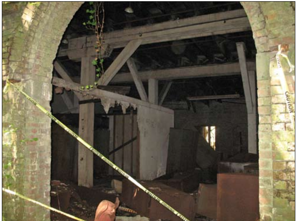
Timber Shed interior 16
