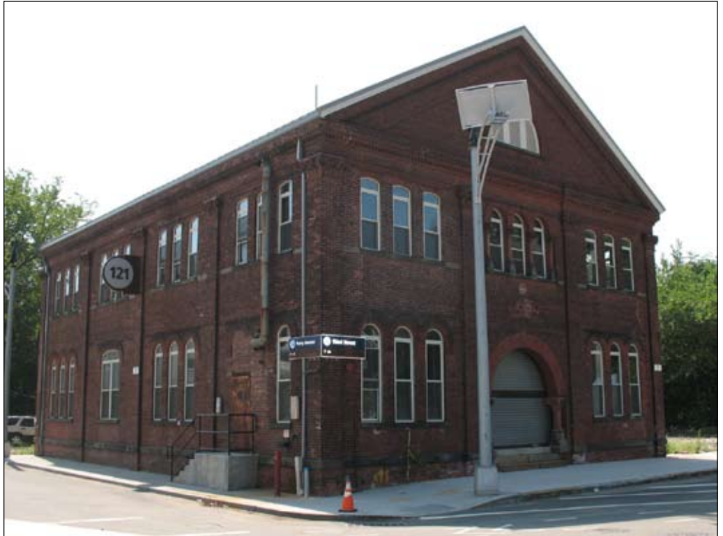
View southeast of Building 121. The Admirals Row site is located behind the building to the south 23
