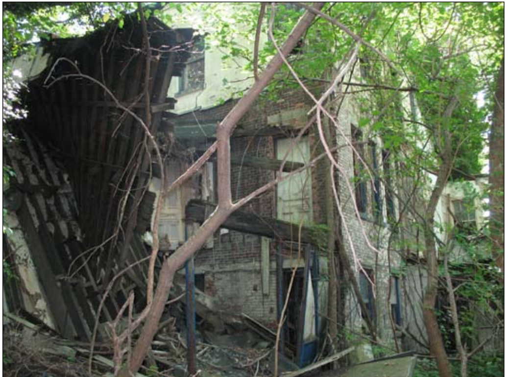
Rear (north) and west facades of Building K 10
