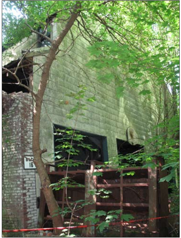
South (Park Street) façade 15
