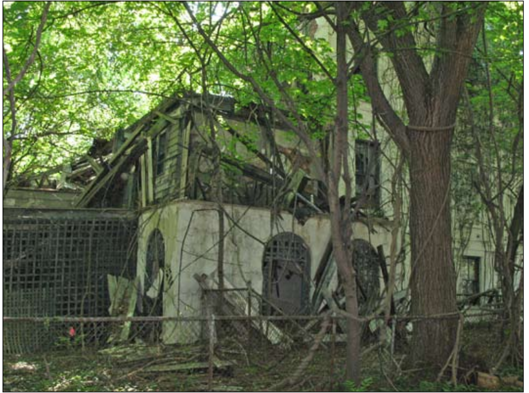
West facade of Building E 7
