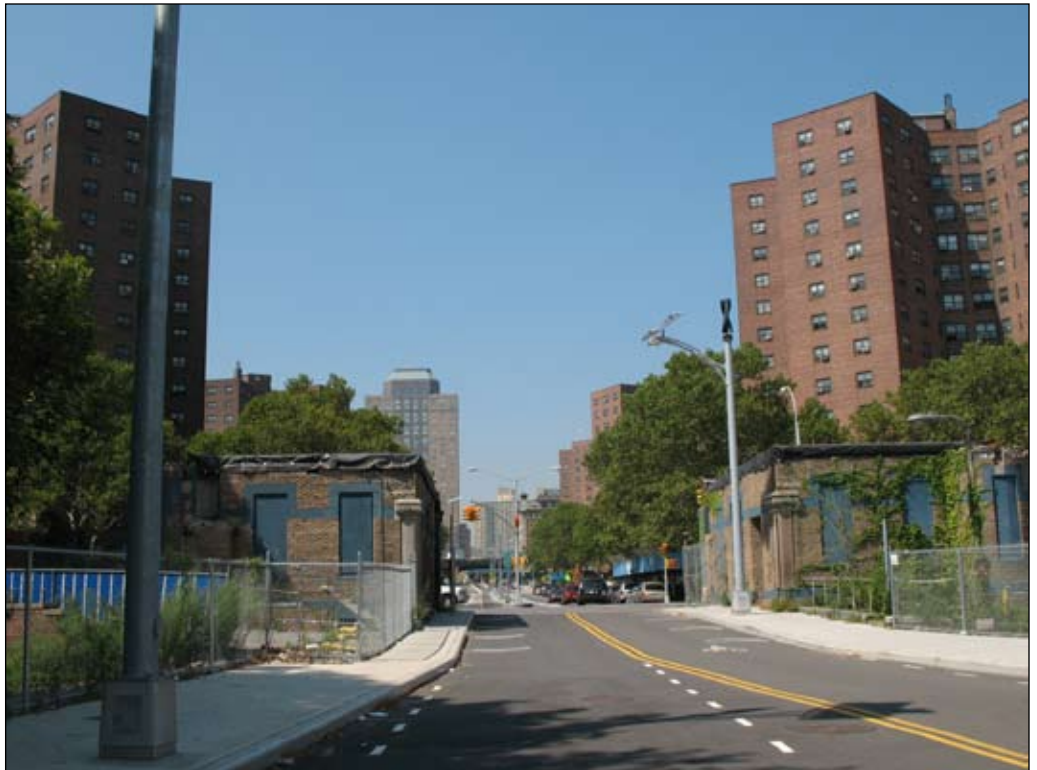
View west to Sands Street Gatehouse structures 26
