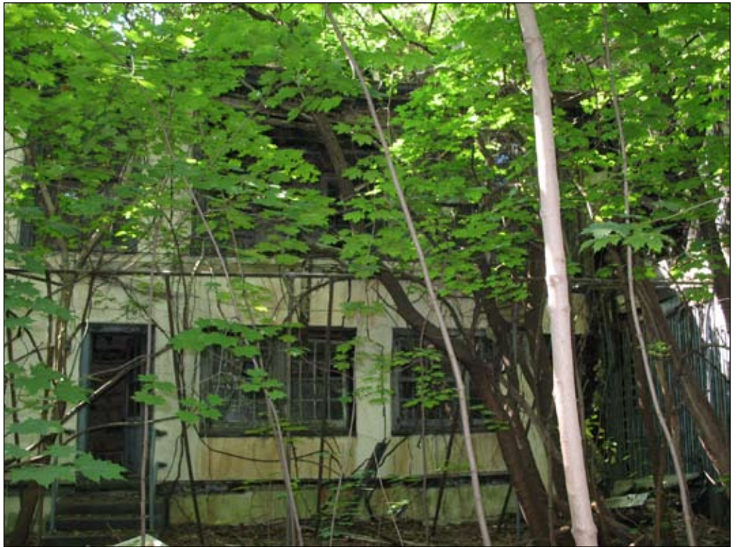
Rear (north) façade of Building G 8
