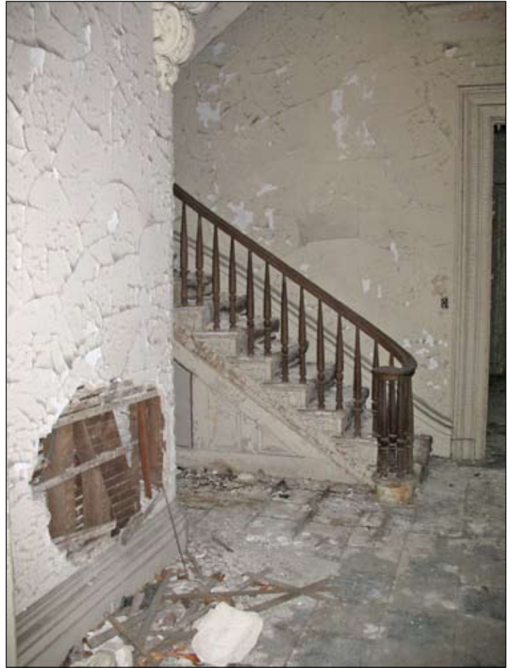
Hall and stairs, first floor 3
