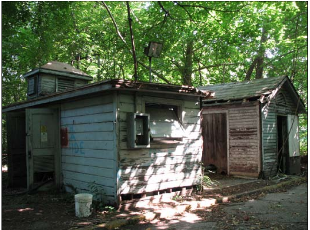
South (Park Street) façade and west façade of the former Building 198 18
