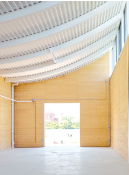
The Lindsay Boathouse, under construction in summer 2023
