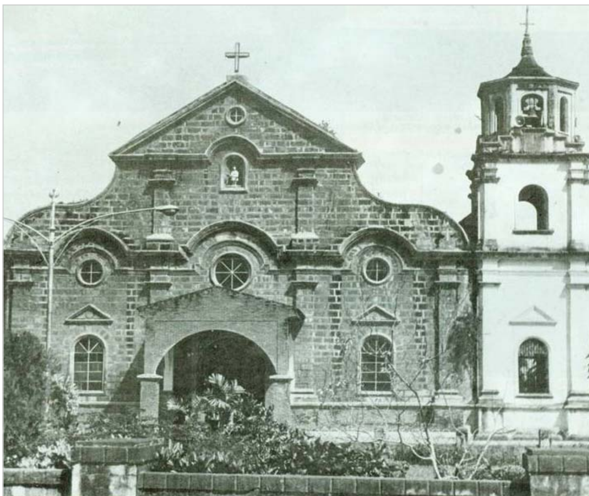
Façade of San Juan Church
