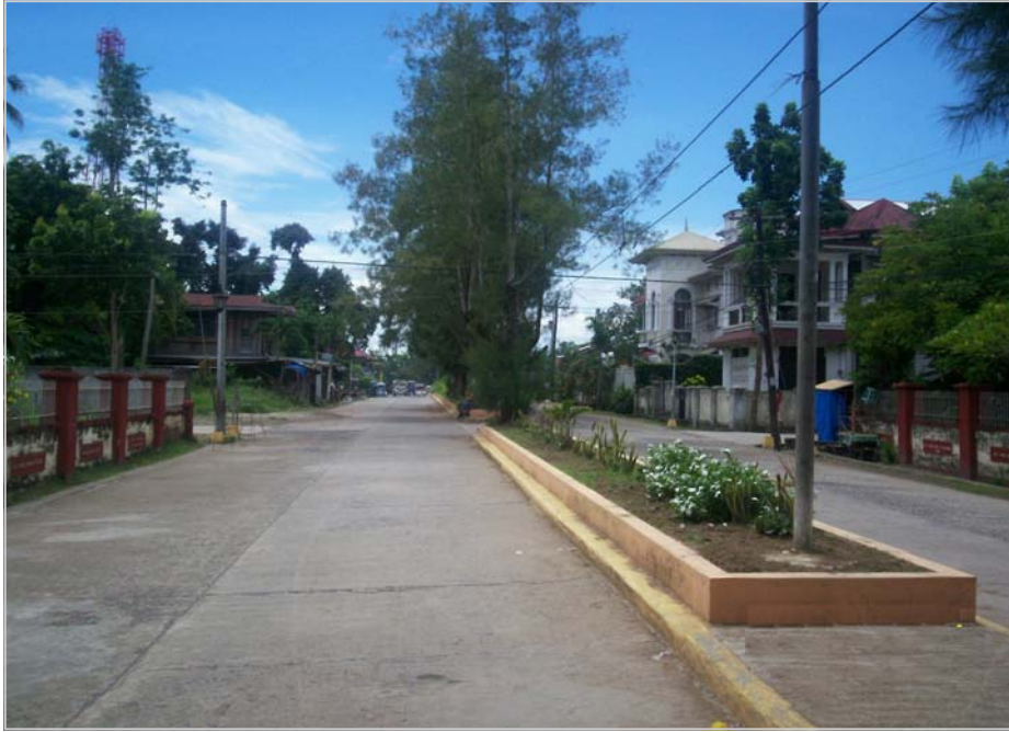
Rizal Street leading to the Calle Mayor and showing the two Triviño heritage houses on its right side. (Source : Mayo, Leon M. Casa Leon : An Ancestral House in San Juan Batangas . 2007)
