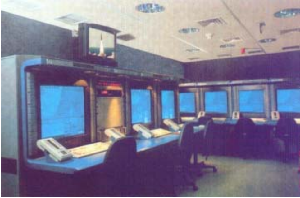
Figure 8 Inside view of the Citron Tree fire Control system (Tadiran 2000) 36
