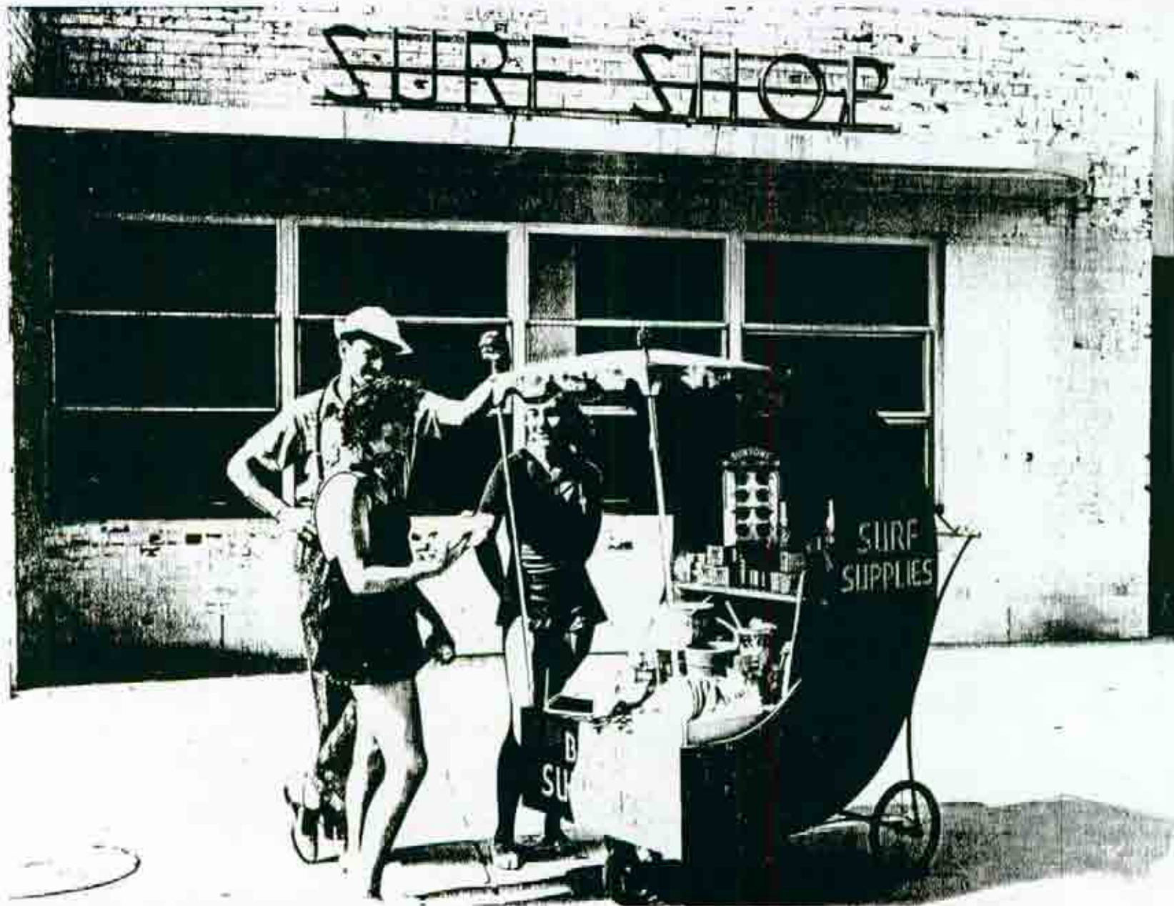
Fig. A-26 Concession area along Promenade at Beach Pavilion (9/15/40)
