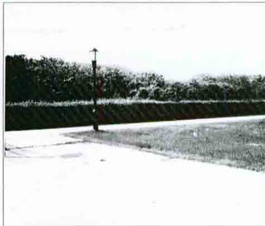
Figure 33: New York Type "B" cast metal light in Bathhouse area
