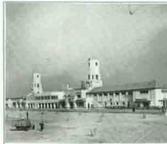
Figure 15: View of Completed Bathhouse, 1939
