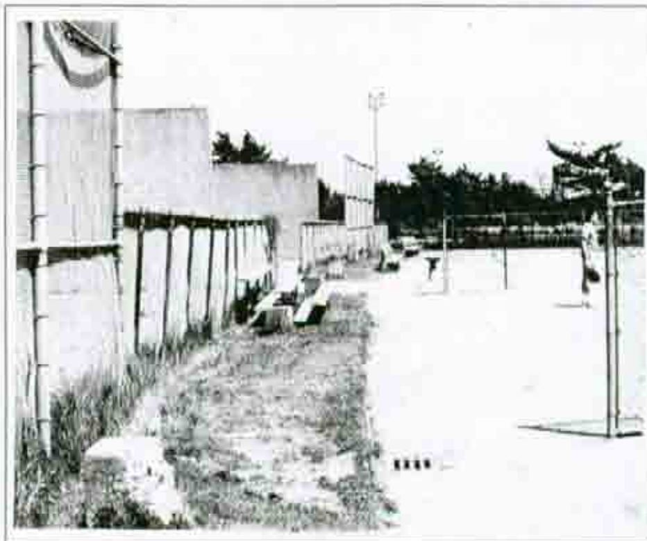
Figure 63: Typical chain link fences in poor repale
