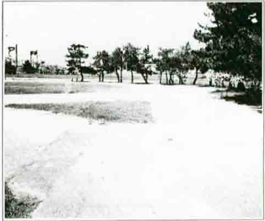
Figure 44: Typical Mall pavement condition
