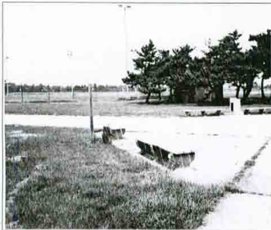
Figure 57: Ballfield electrical hut
