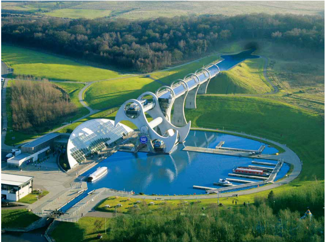
Aerial view of the Falkirk Wheel, 2018 © Scottish Canals
