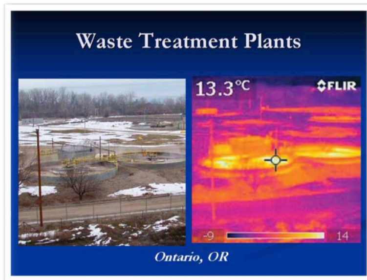
Numerous sensors are located at waste treatment plants. An infrared image of the scene shows the output of heat from the waste treatment beds right next to the sensor. (Photos by Anthony Watts, surfacestations.org .)
