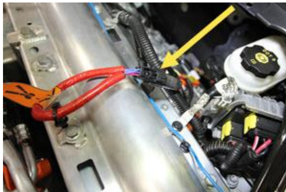
Figure 15. Disconnecting the First Responder Loop
