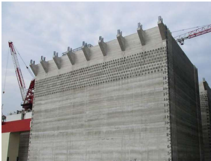
Figure 14: Caissons with roughed surface to promote coral growth
