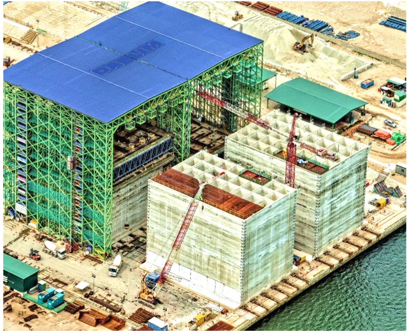
Figure 7: Typical caisson structure
