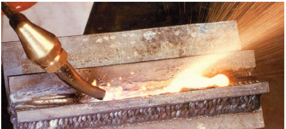
Figure 14. Oxy-acetylene gouging application
