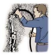
**FIG. 7** - Moistening the area to be repaired prevents the newly applied patch from drying out.
