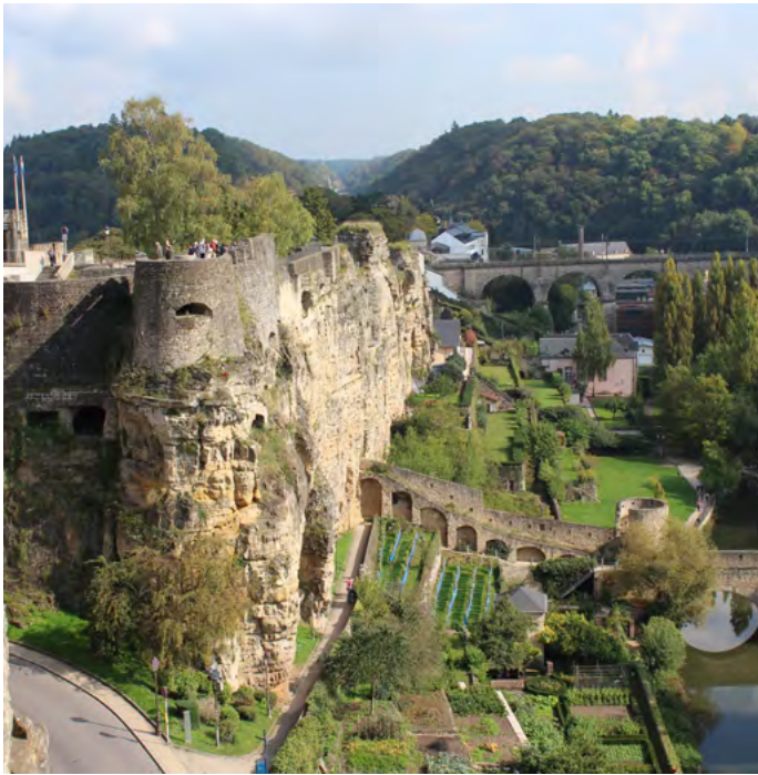
The location of the "small castle" that was first called "Luxembourg" at the end of the 10th century © SIP
