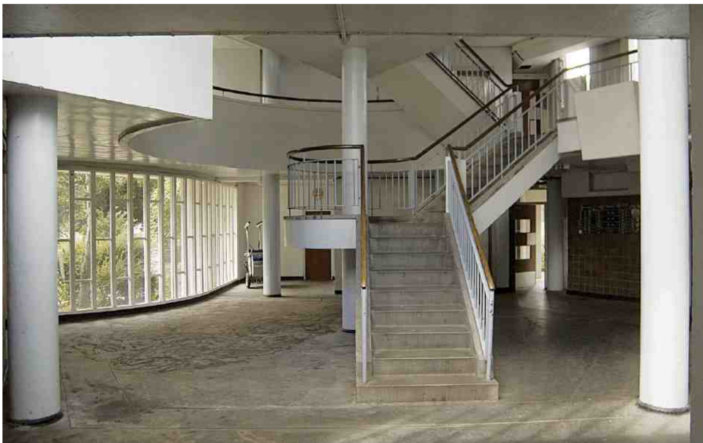
312. Bevin Court, base of stair in 2007
