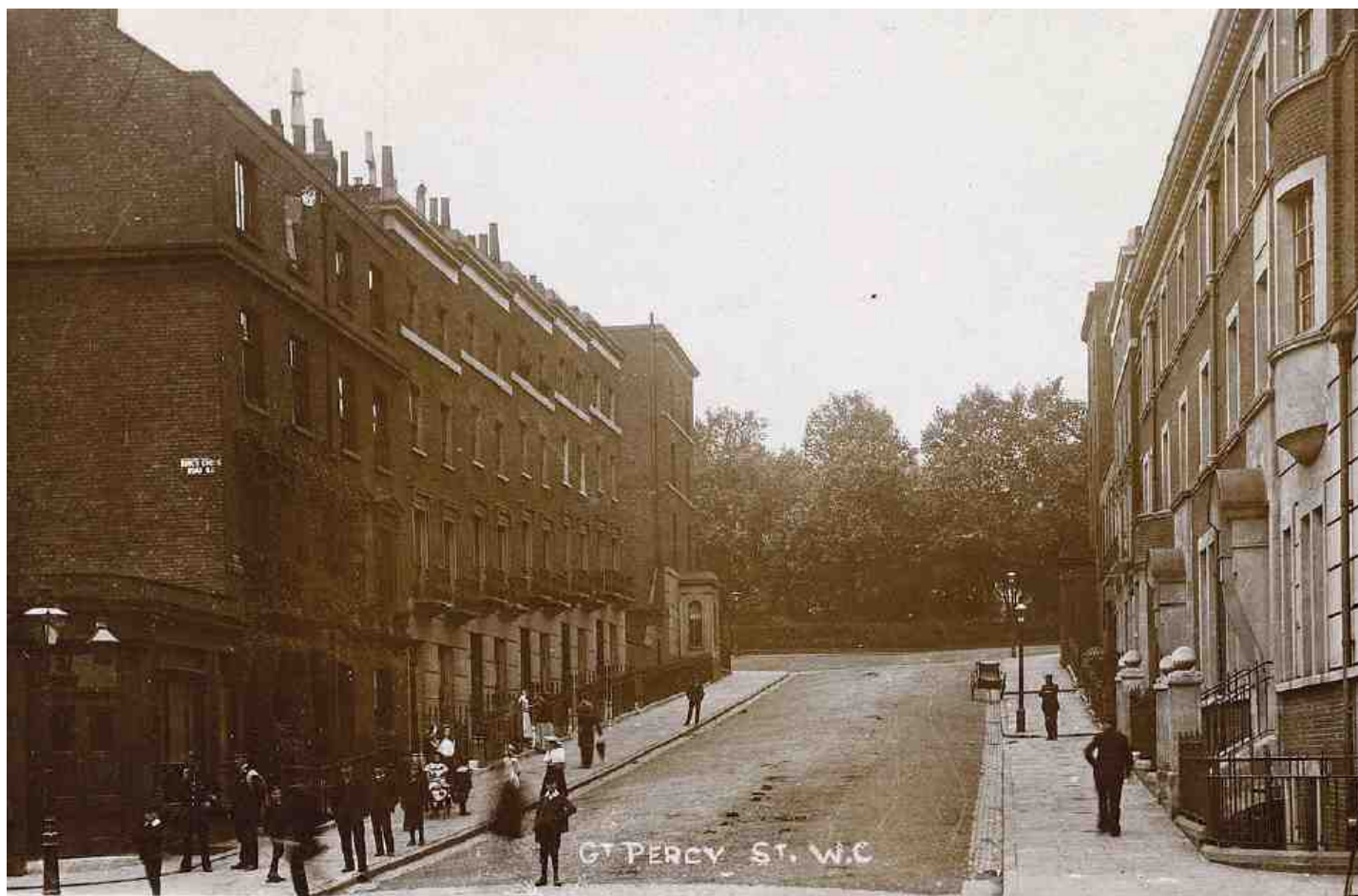
290. Great Percy Street, lower section, looking east to Percy Circus in 1906. Left, Nos 1–13, built 1844–53 ( demolished ); right, flank of Clerkenwell Police Court, King's Cross Road
