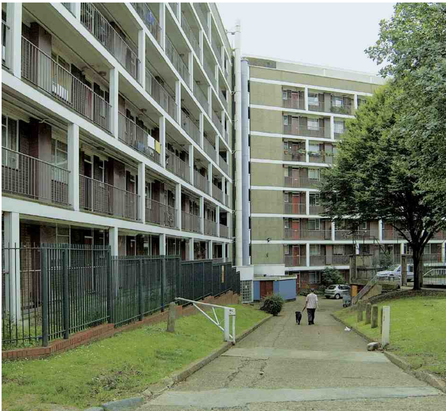
309. Rear (north-east) front in 2007 showing galleries to flats
