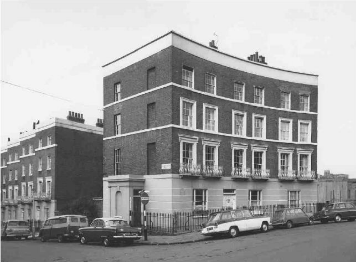
292. Nos 16–18 Percy Circus in 1965. Nos 7–13 Great Percy Street to left. All demolished
