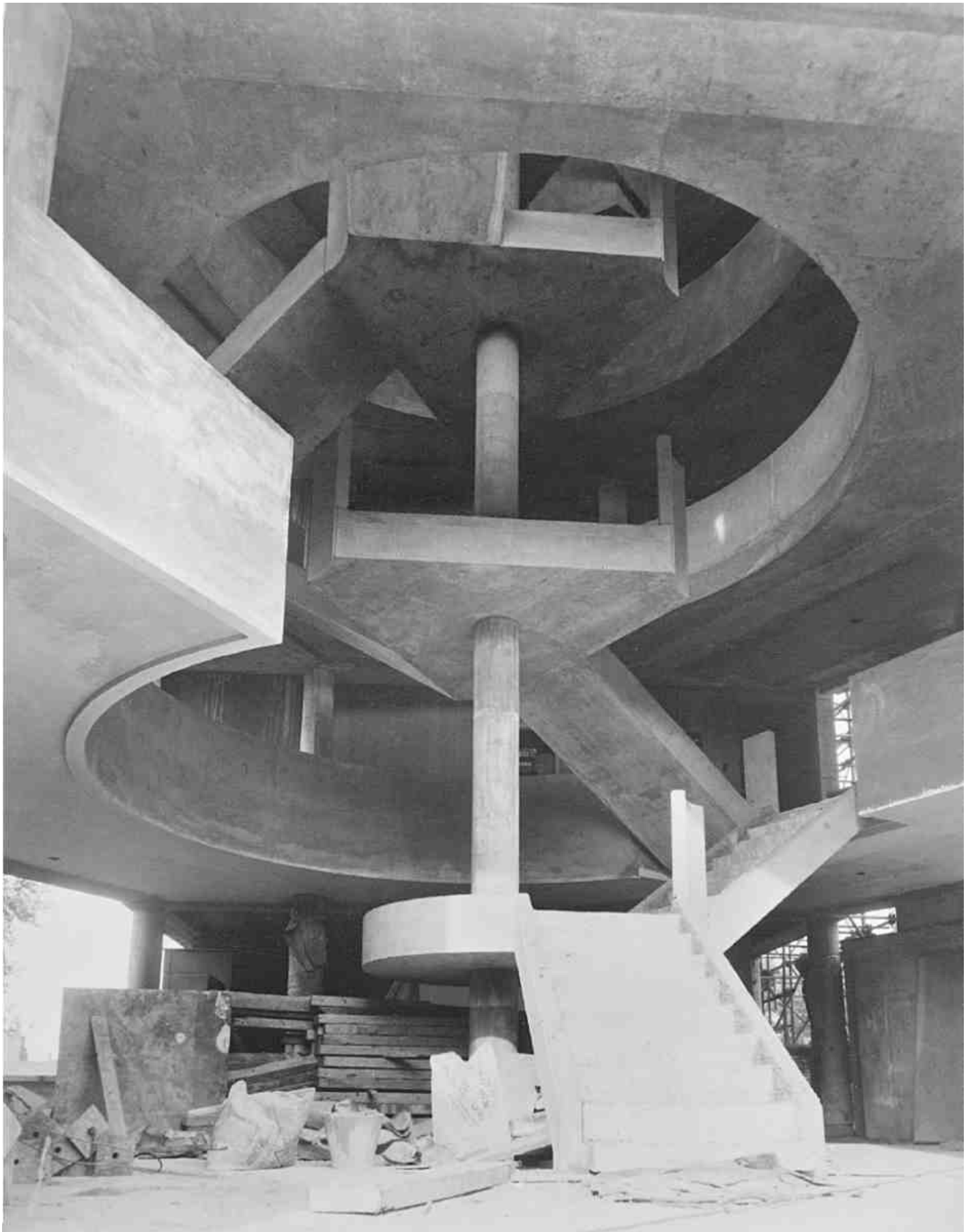
311. Bevin Court staircase, during construction, c. 1952
