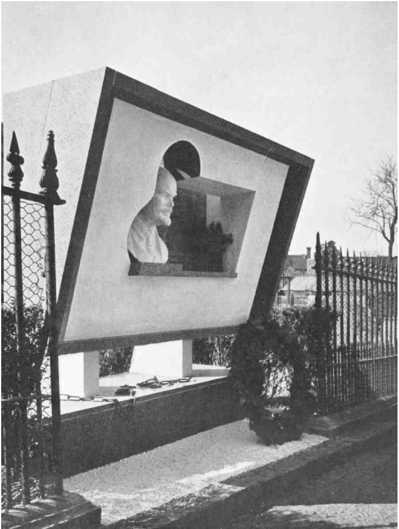
301. Lenin Memorial, between railings facing No. 30 Holford Square. Designed by Berthold Lubetkin for Finsbury Council, 1942. Demolished
