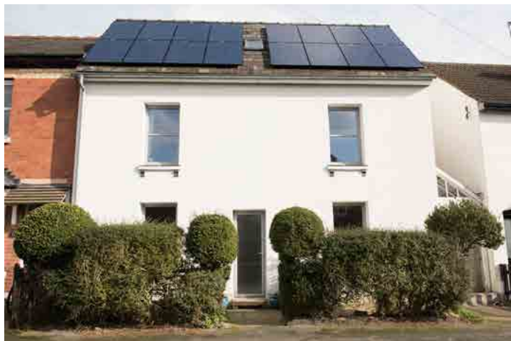
An Ecology-backed Passivhaus EnerPHit renovation
