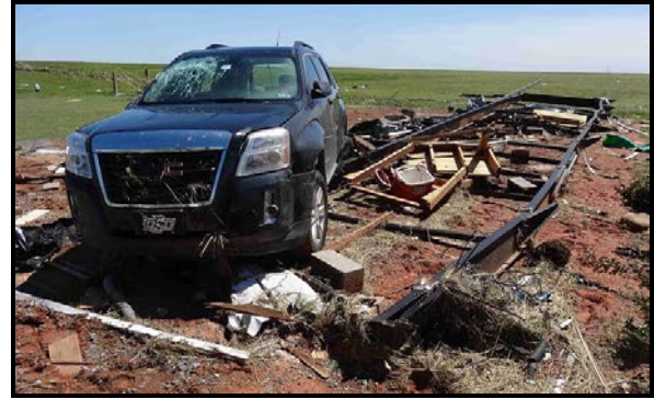
Figure 14. An SUV that came to rest on the steel frame of a destroyed single-wide mobile home.
