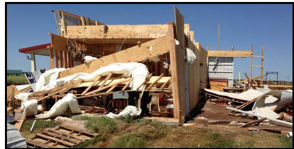
Figure 11. EF1 damage to a metal-clad, wood-framed outbuilding (DoD 6).
