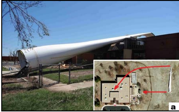
Figure 25. 60m long wind turbine blade that was on display was lifted from its mooring and deposited on a school building to the west. The inset a) image shows the location of the turbine blade before the tornado. Red arrows indicate how the blade pivoted counterclockwise to the west.
