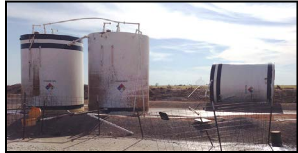
Figure 20. Damage to an oil tank battery near South Country Club Road and 15 th Street Southwest.
