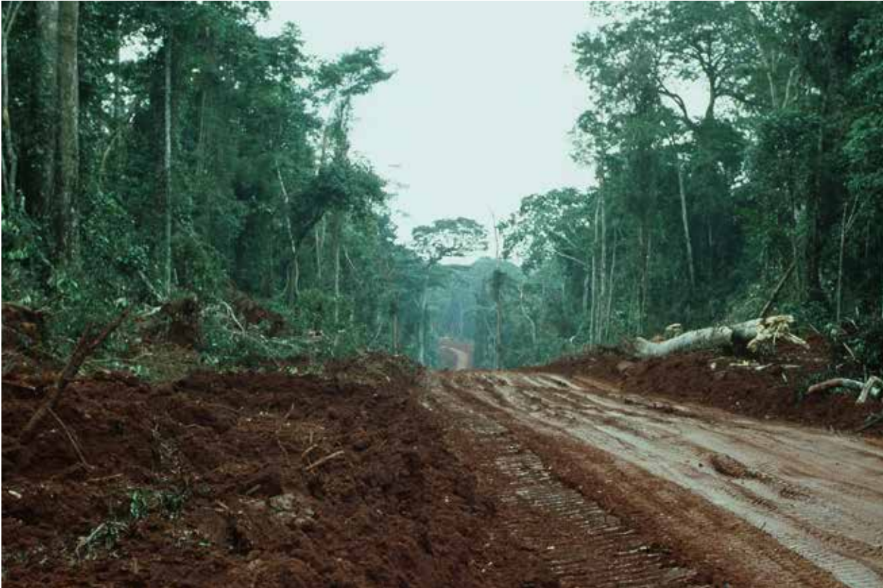
New logging road in east Cameroon. © Greenpeace / Filip Verbelan
