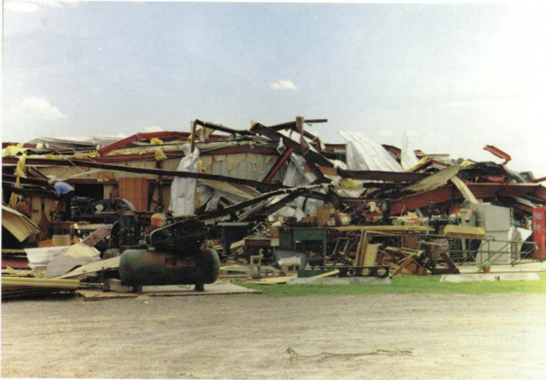
Figure 36. Steel Building Failure
