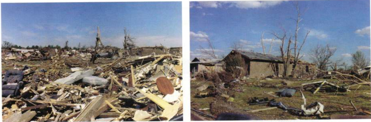
Debris comparison between locations at the middle of the tornado path (left) and locations at the perimeter of the damage path (right).
