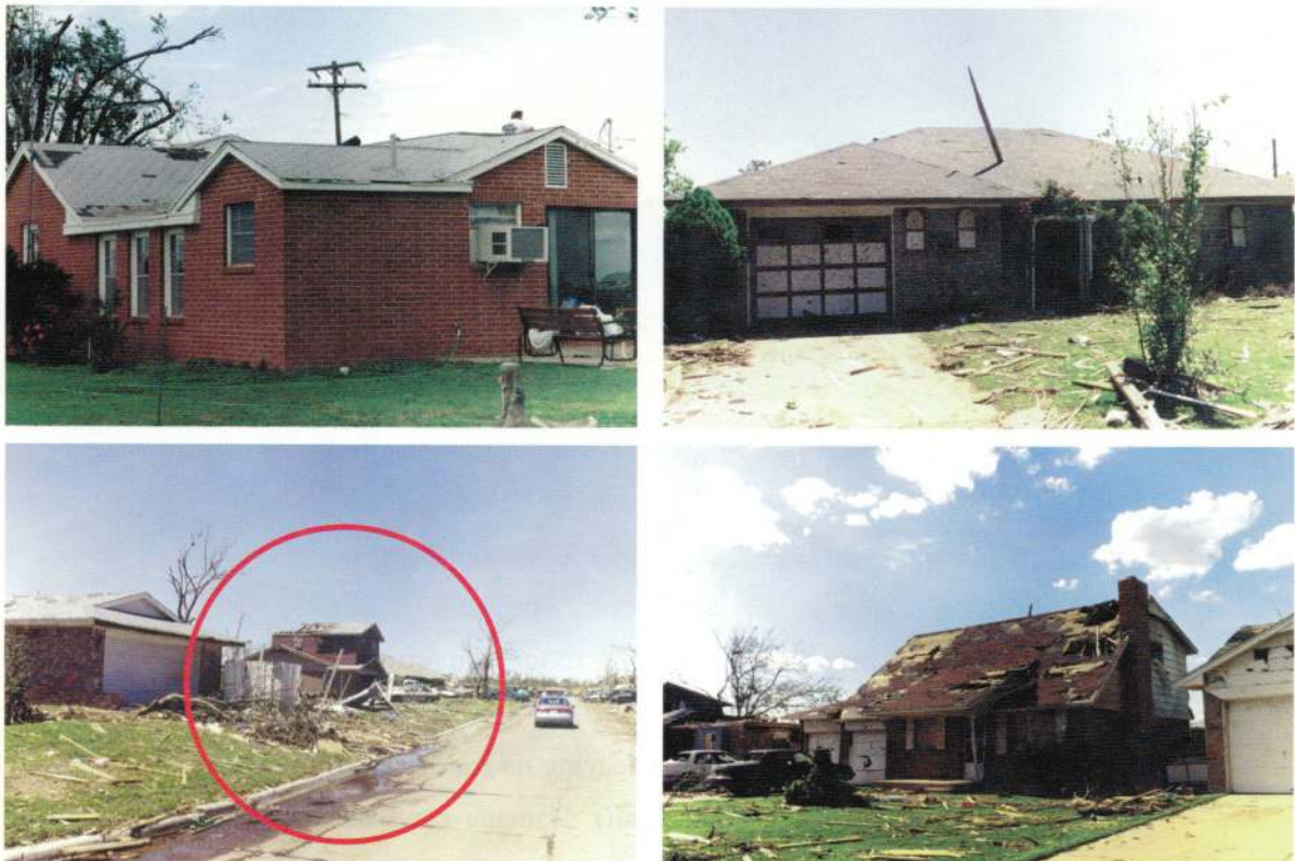
FIGURE 6. MINOR/MODERATE DAMAGE (F0-F1 DAMAGE LEVEL)
