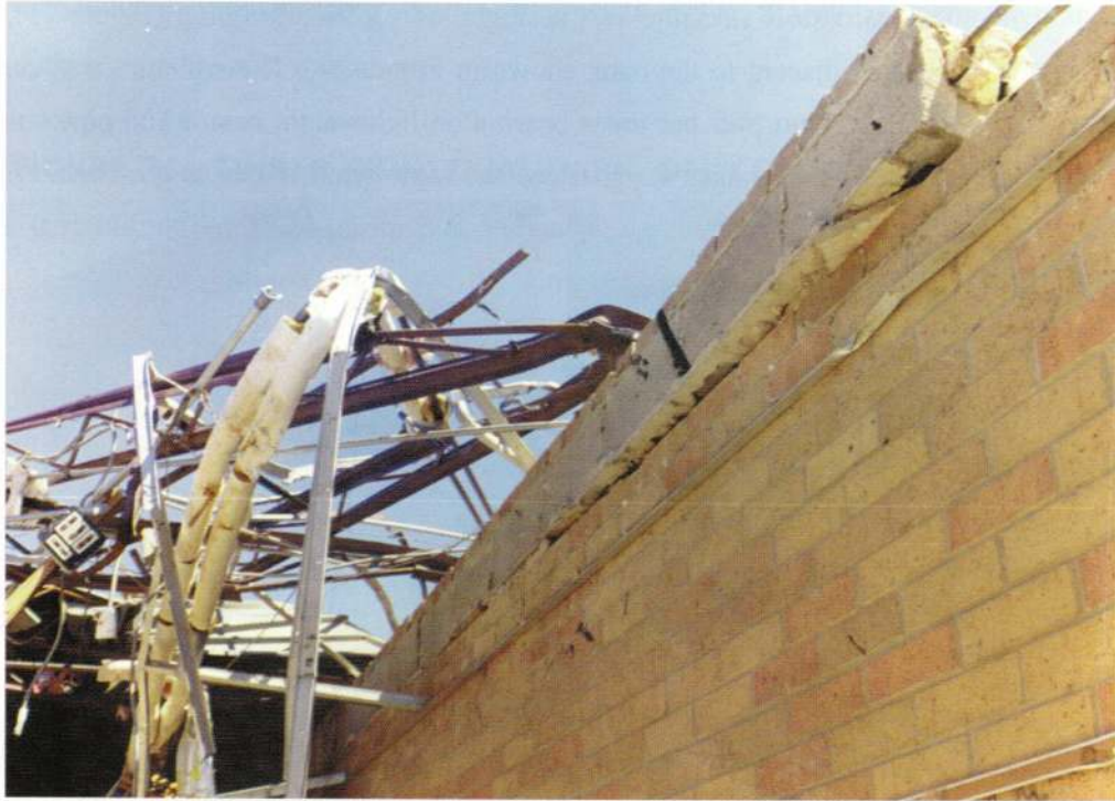
FIGURE 23. KELLY ELEMENTARY, MASONRY BEARING WALL
