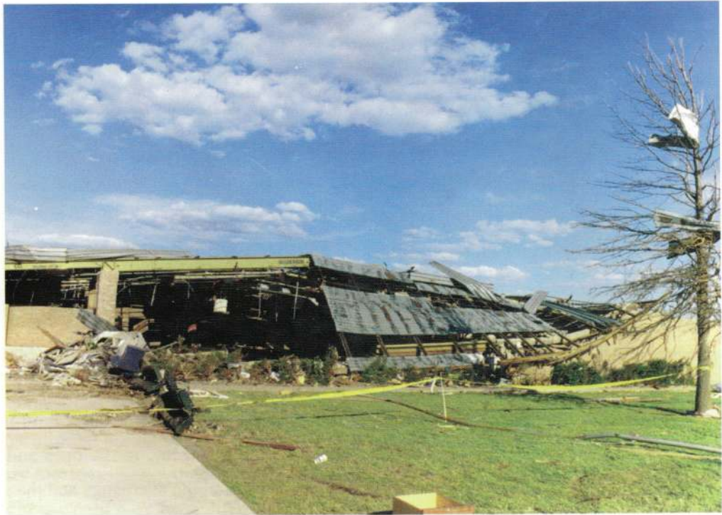
FIGURE 21. KELLY ELEMENTARY SCHOOL, MOORE, OK
