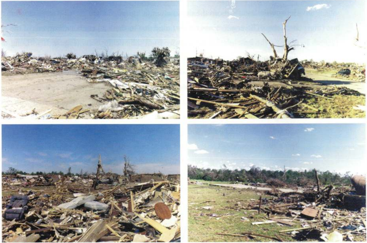
FIGURE 9. DESTROYED (F4-F5 DAMAGE LEVEL)
