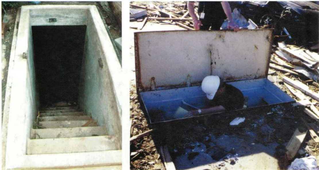
Cast-in-place concrete (left); prefabricated steel (right).
