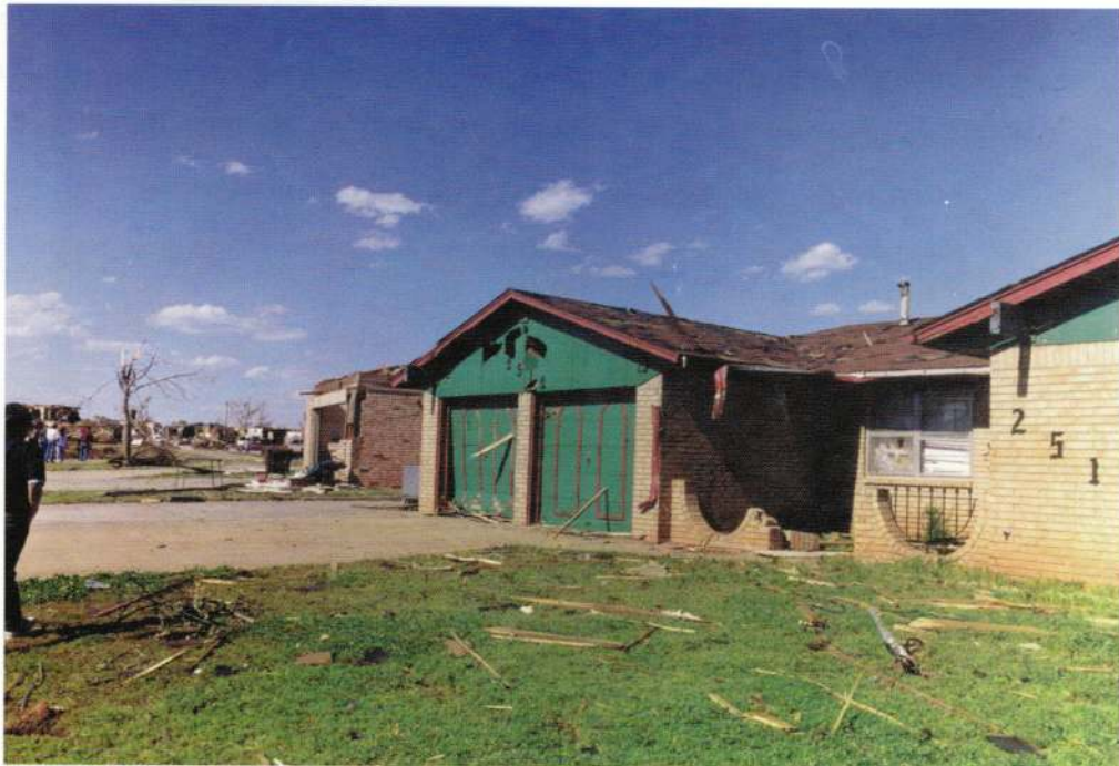
FIGURE 4. GARAGE DOOR DAMAGE
