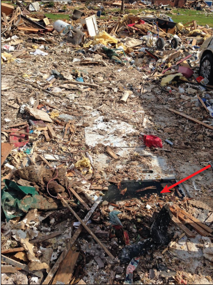
Figure 9. Observation 7: Below-ground shelter in a heavily damaged area (red arrow indicates entrance) (Oklahoma City, OK)
