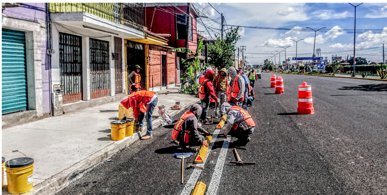
Photo 6-2: Installation of a protected cycle lane in Cholula, Mexico.
