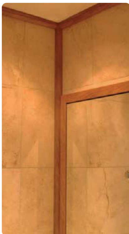
pic D-Line 30x30mm ¼ Round Trunking as coving/cornice. Reducing Tee connects to 30x15mm Mini Trunking for lighting & smoke alarm cables. Ref Social Housing rewires
