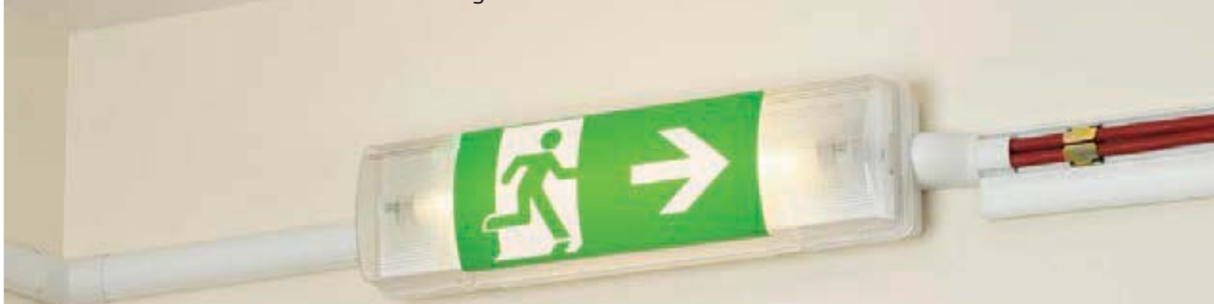
Pic shows SAFE-D30 in D-Line Mini Trunking 30x15mm
