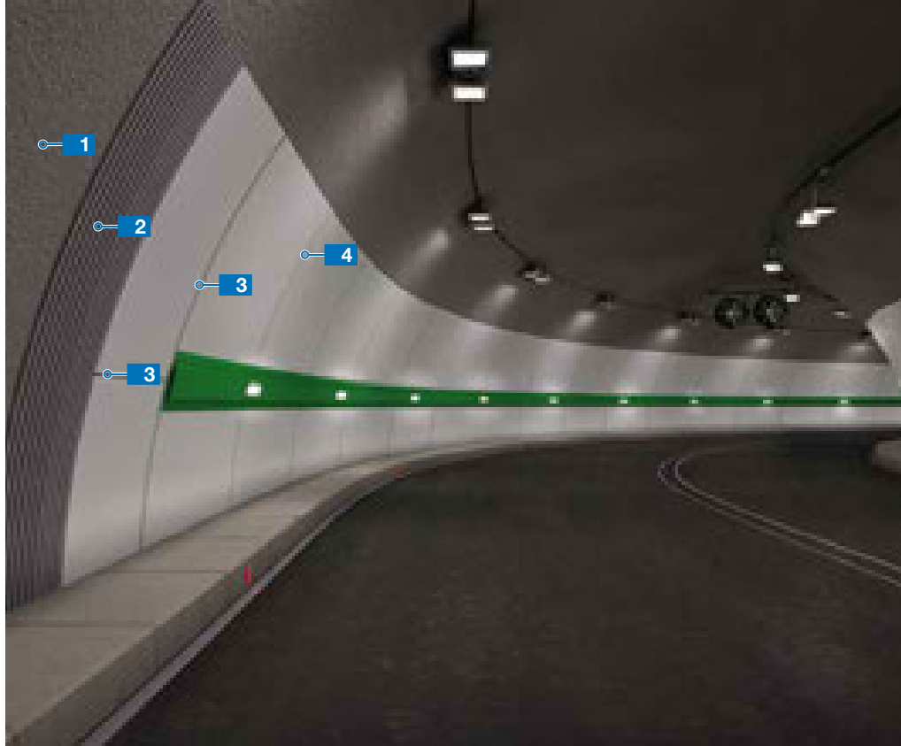
Sistema per la posa di rivestimento in ceramica in galleria System for the installation of ceramic tiles in tunnels
