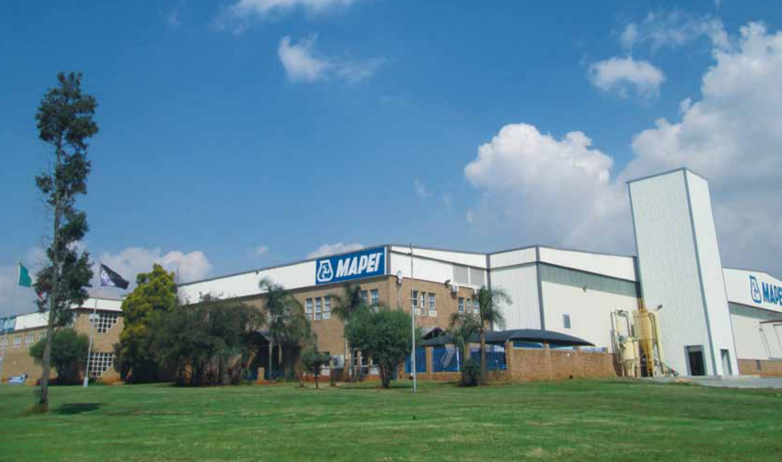
The MAPEI Facility in Roodekop, Germiston
