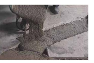
Castable quick-setting and hardening, shrinkage compensated, high-ductility mortar with rigid metallic fibres. Suitable for application down to -5°C.
