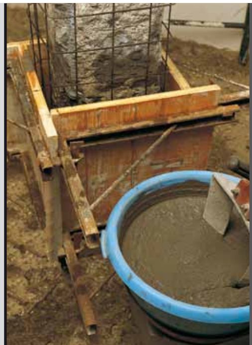
photo 10 Structure repaired using Mapegrout HI-FLOW
