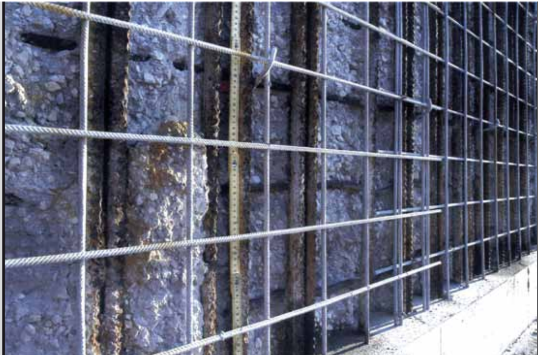
photo 4 Positioning new reinforcement
