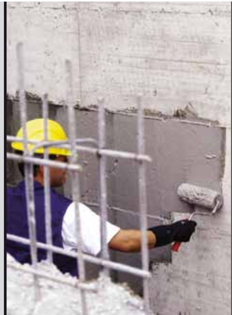
photo 16 Mapelastik Smart applied with a roller
