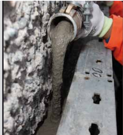
photo 11 Application of Mapegrout HI-FLOW GF
