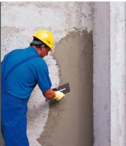
photo 18 Smoothing layer using Monofinish
