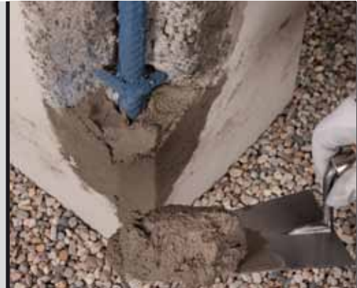
photo 9 Application of MAPEGROUT LM2K
