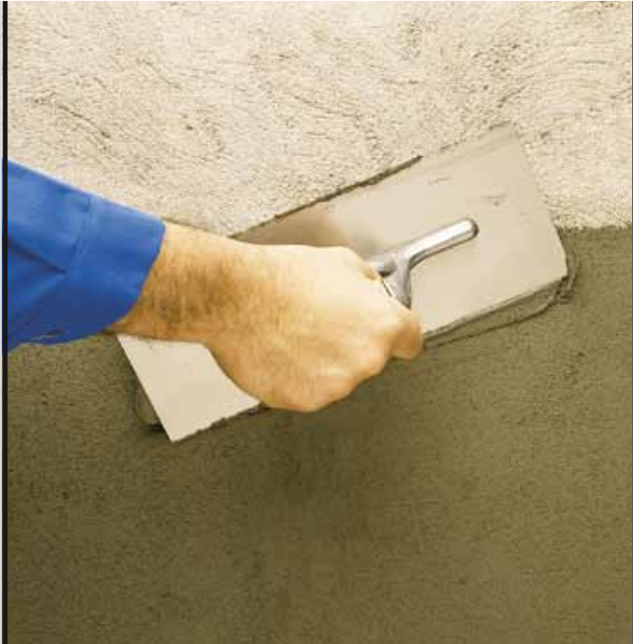
photo 17 Smoothing layer using Mapefinish
