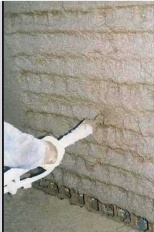
photo 5 Mapegrout Easy Flow applied by spray
