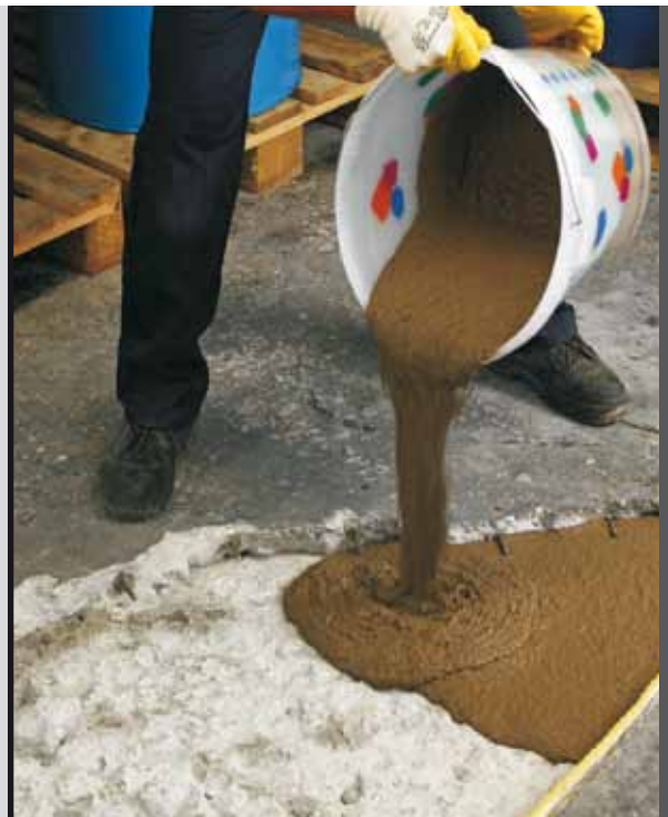
photo 13 Repairing a floor using Mapegrout SV Fiber
