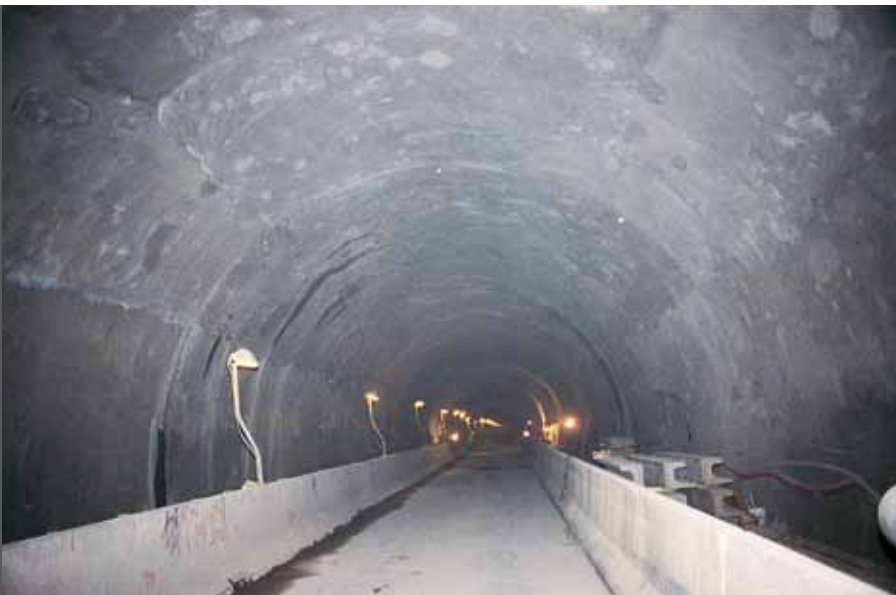
photo 6 Structure repaired using Mapegrout T60
