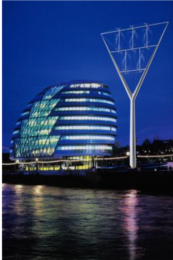
Figure 36. The Beacon: a conceptual design of vertical wind turbines providing power for green buildings.
