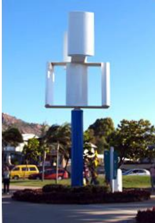
Figure 12. Hybrid Darrieus and Savonius Ropatec vertical axis wind generator.
