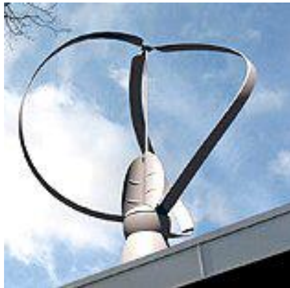
Figure 2. Hybrid Darrieus and Savonius self-starting Neoga turbine on top of a building.
