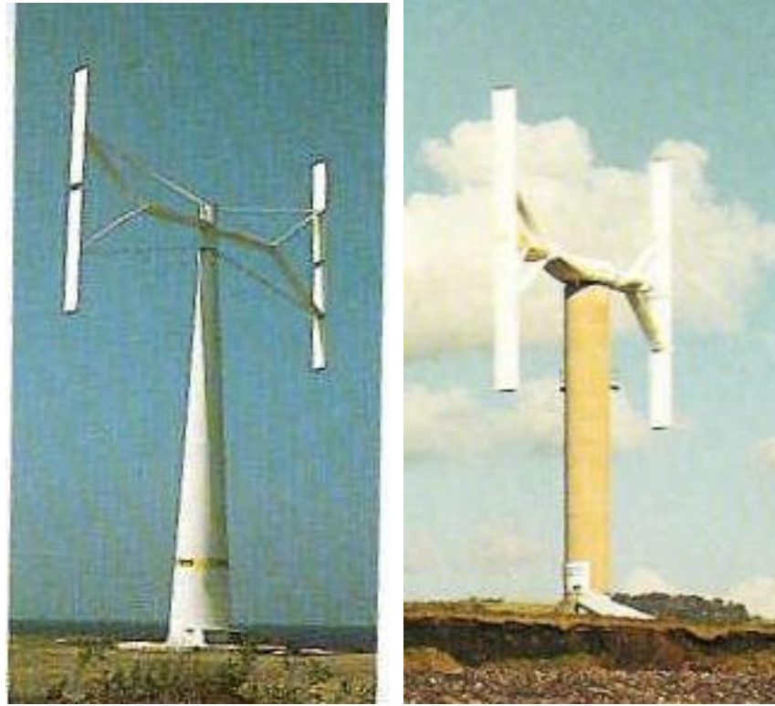
Figure 7. Variable Geometry wind turbine machines.
