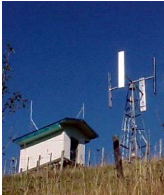
Figure 15. Four rotor vertical axis wind generator for remote sites.
