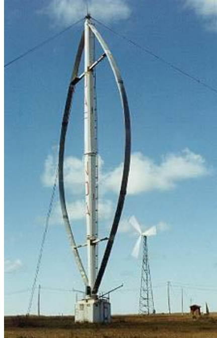
Figure 1. Darrieus vertical wind turbine with the generator positioned at the base of the tower. The tower is reinforced with guy wires.
