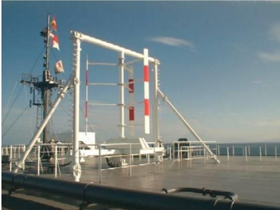
Figure 19. Vertical axis wind turbine in a marine environment.
