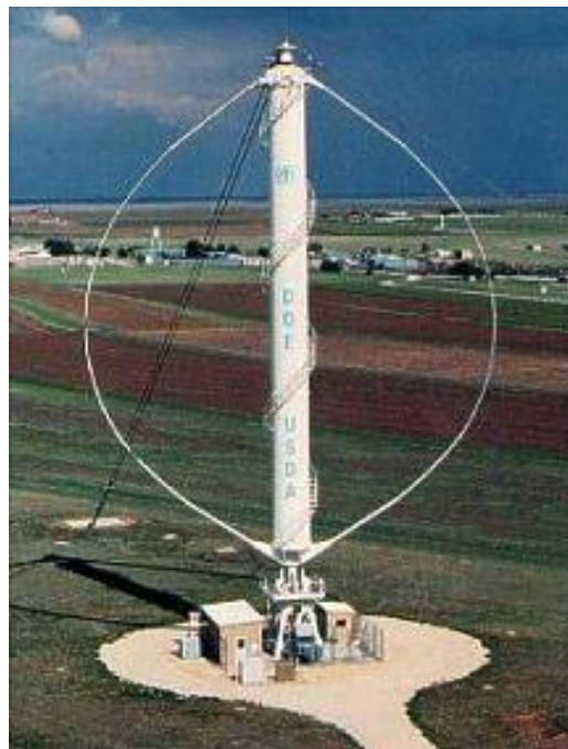
Figure 5. Experimental Department of Energy (DOE) and US Department of Agriculture (USDA) 34 meter diameter Darrieus wind turbine.
