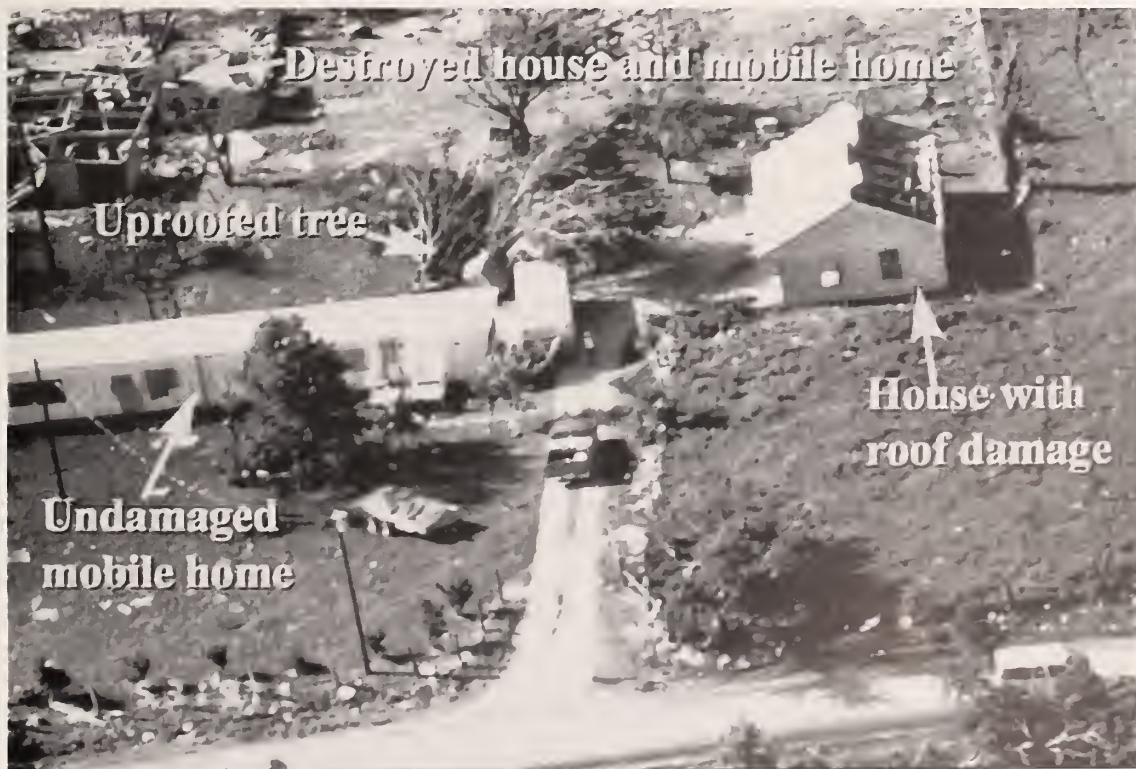
Figure 14. Structural damage near the end of the path of the Jarrel tornado.
