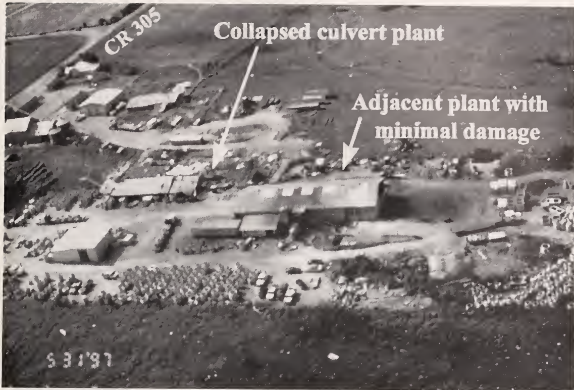
Figure 8. Aerial view of entire culvert plant complex.
