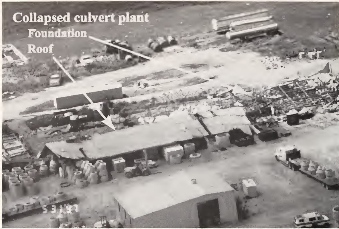
Figure 6. Aerial view of collapsed culvert plant.
