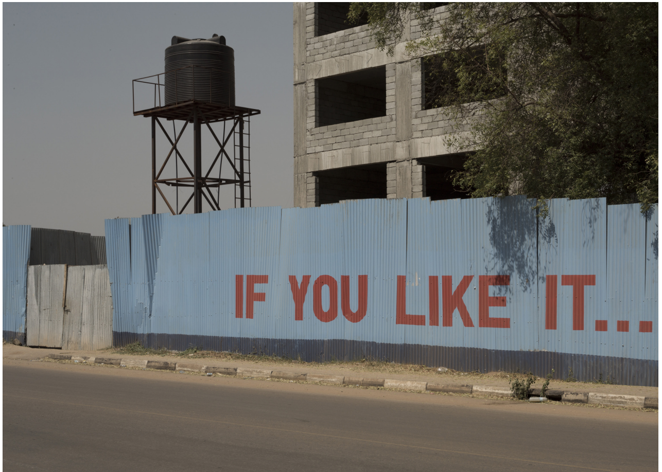
L1000125. Construction site / Hai Jalaba District / Juba / 2015
