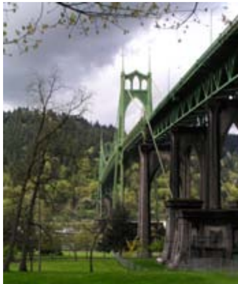
The St. Johns Bridge, built in 1931, underwent a major rehabilitation from 2003 to 2006.
