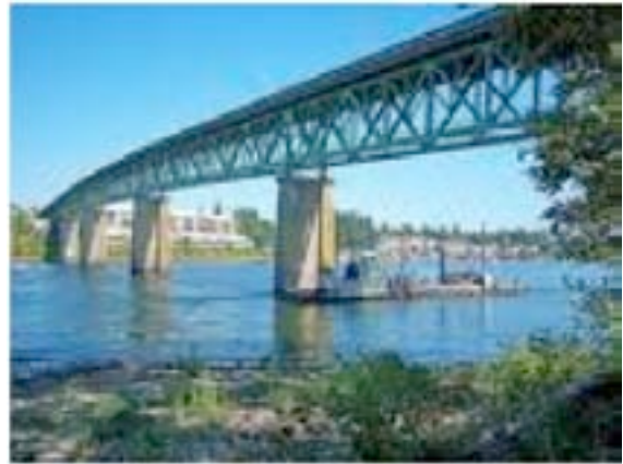
The Sellwood Bridge over the Willamette River is ranked as the least safe bridge in Multnomah County with a sufficiency rating of 2 out of 100.
