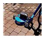
Re-sealing your pavers may be necessary on a regular basis to maintain color and appearance. It also helps protect the pavers against stains, algae and loss of joint sand.
