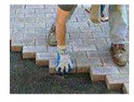
into the paver design. If pavers need to be cut to size, use a diamond saw, masonry chisel or mechanical splitter and safety glasses.
