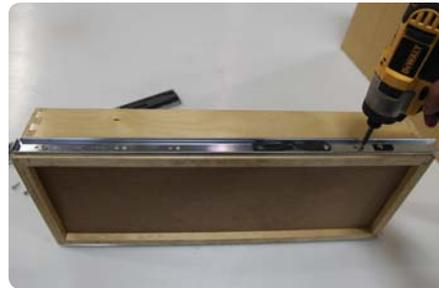
Locate the small drawer box slide, and using two screws (A), fasten it to the drawer box as shown.
