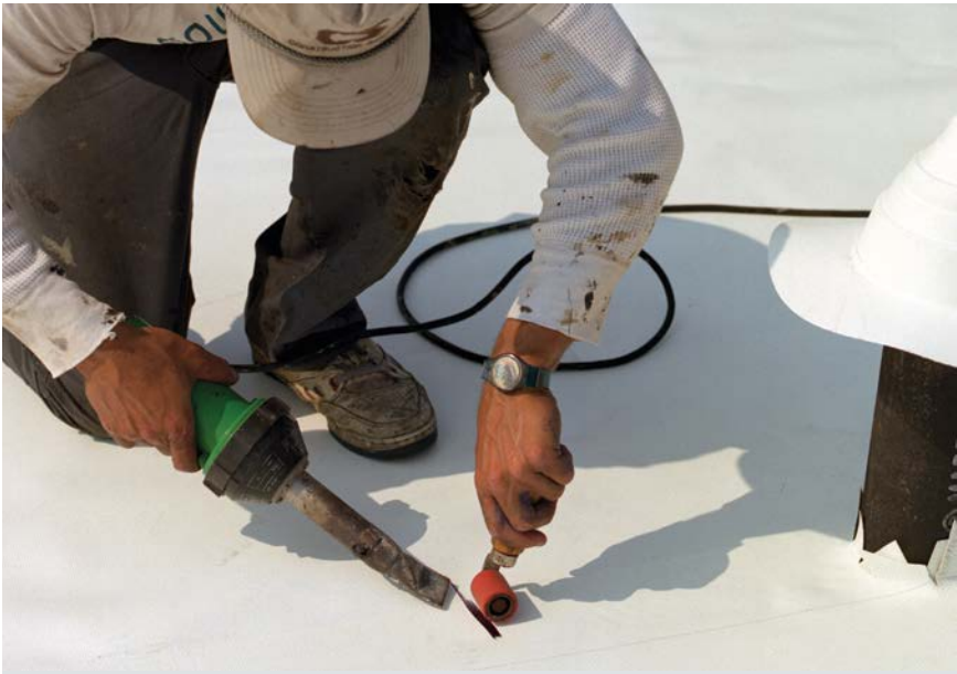
Cool roofs can be made of either white or darker colored materials. While white roofs are usually cooler, both will reflect near-infrared sunlight and save energy and money.
