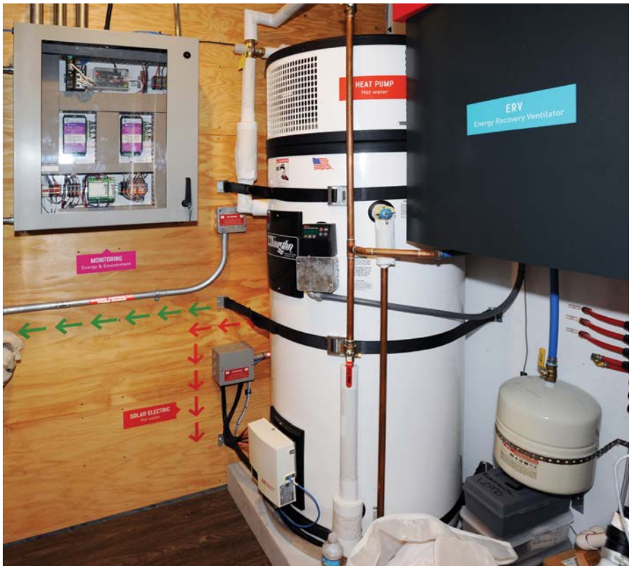
If you're in a climate where temperatures are 40°–90°F all year, consider a heat pump water heater to cut water heating costs by 50%.
