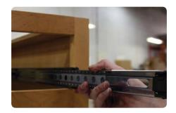
Check that the slide is both level, and parallel to the cabinet. Mark the back of the cabinet, and drill 2 .0625" diameter pilot holes.
