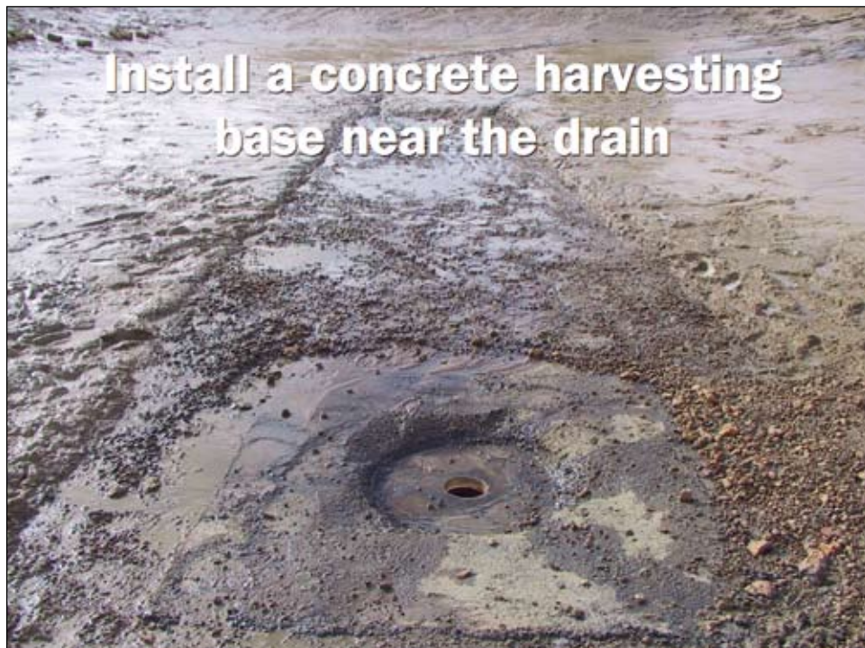
Slide 14. Install a concrete harvesting base near the drain.
