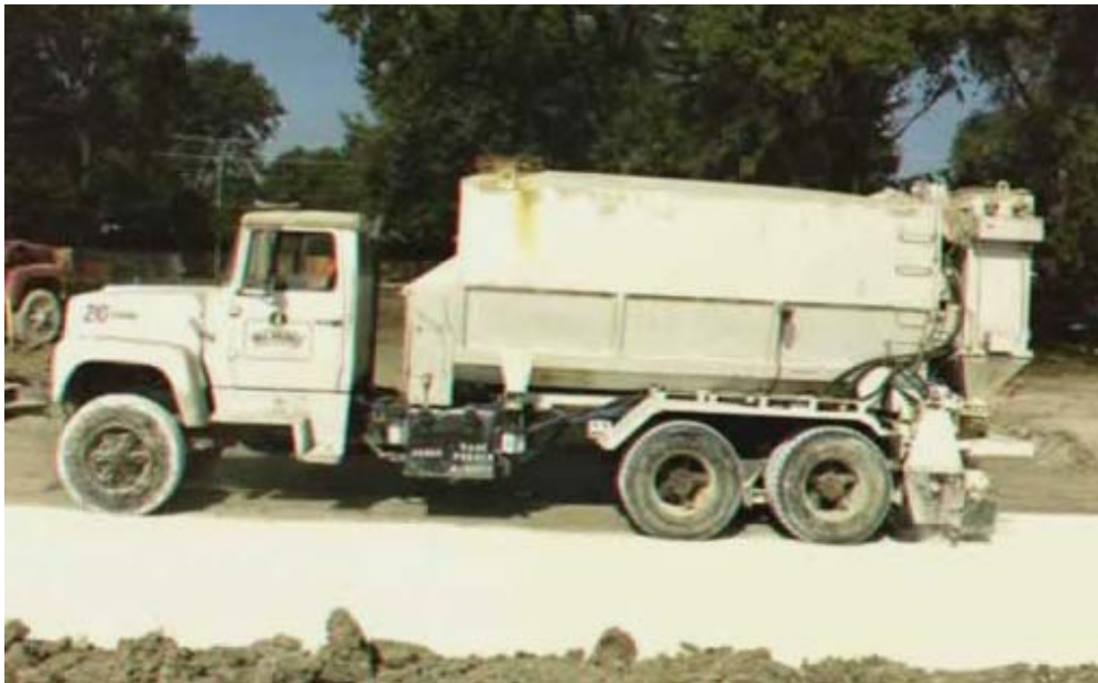
Figure 10: Dry lime application with mechanical spreader 4
