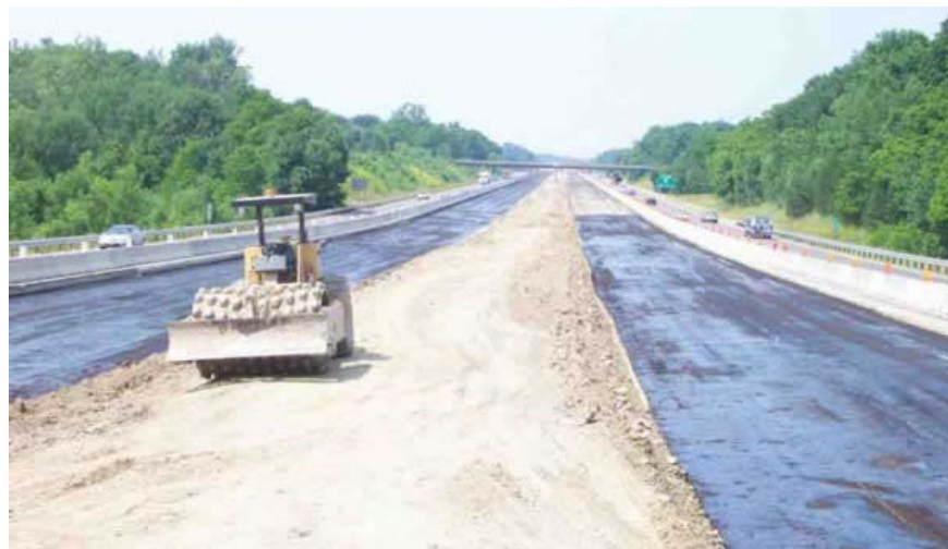
Figure 19: Prime coat emulsion for curing
