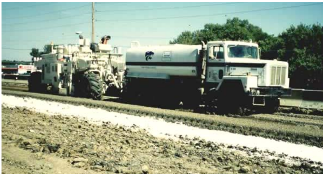
Figure 15: Rotary mixer with water truck attached
