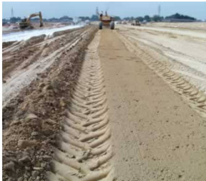
Figure 16: Mixing and pulverization
