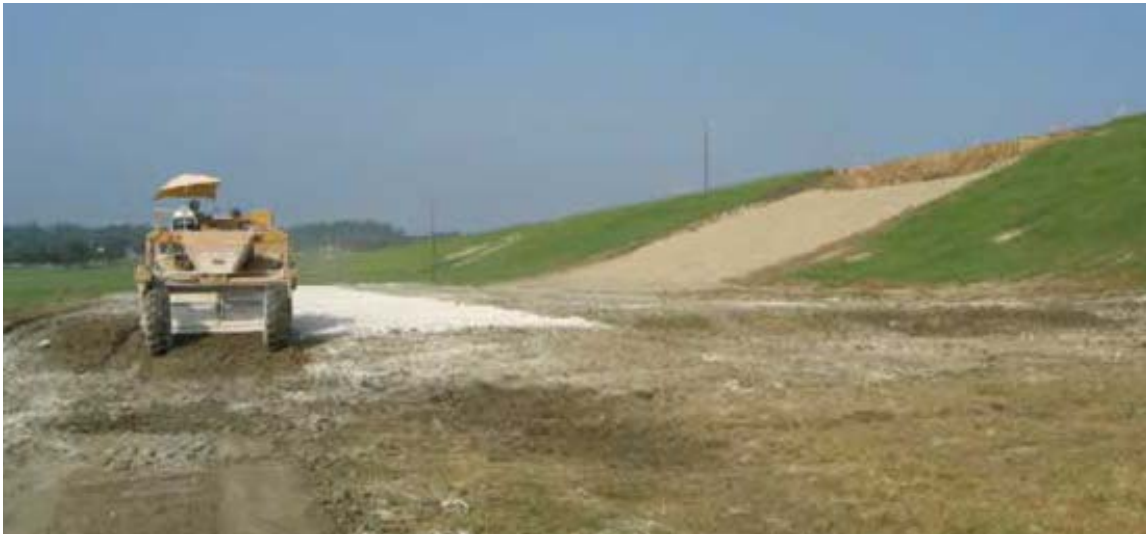
Figure 23: Preliminary mixing of lime and embankment soils in mixing area
