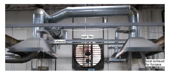
Figure 5: Wall fan and canopy hoods in the post-treatment area.
