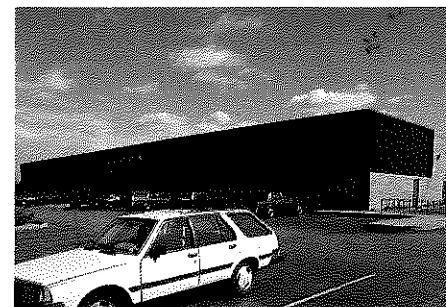
Four Seasons Brunswick Bowling, located in Chesterfield, Missouri.
