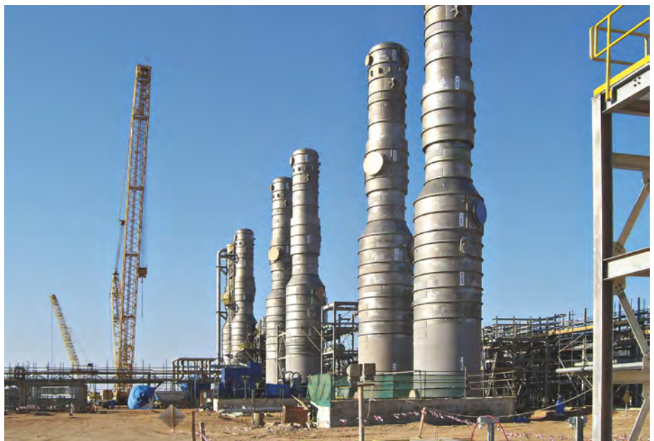
2507 stainless steel enhanced oil recovery equipment. © Aquatech
