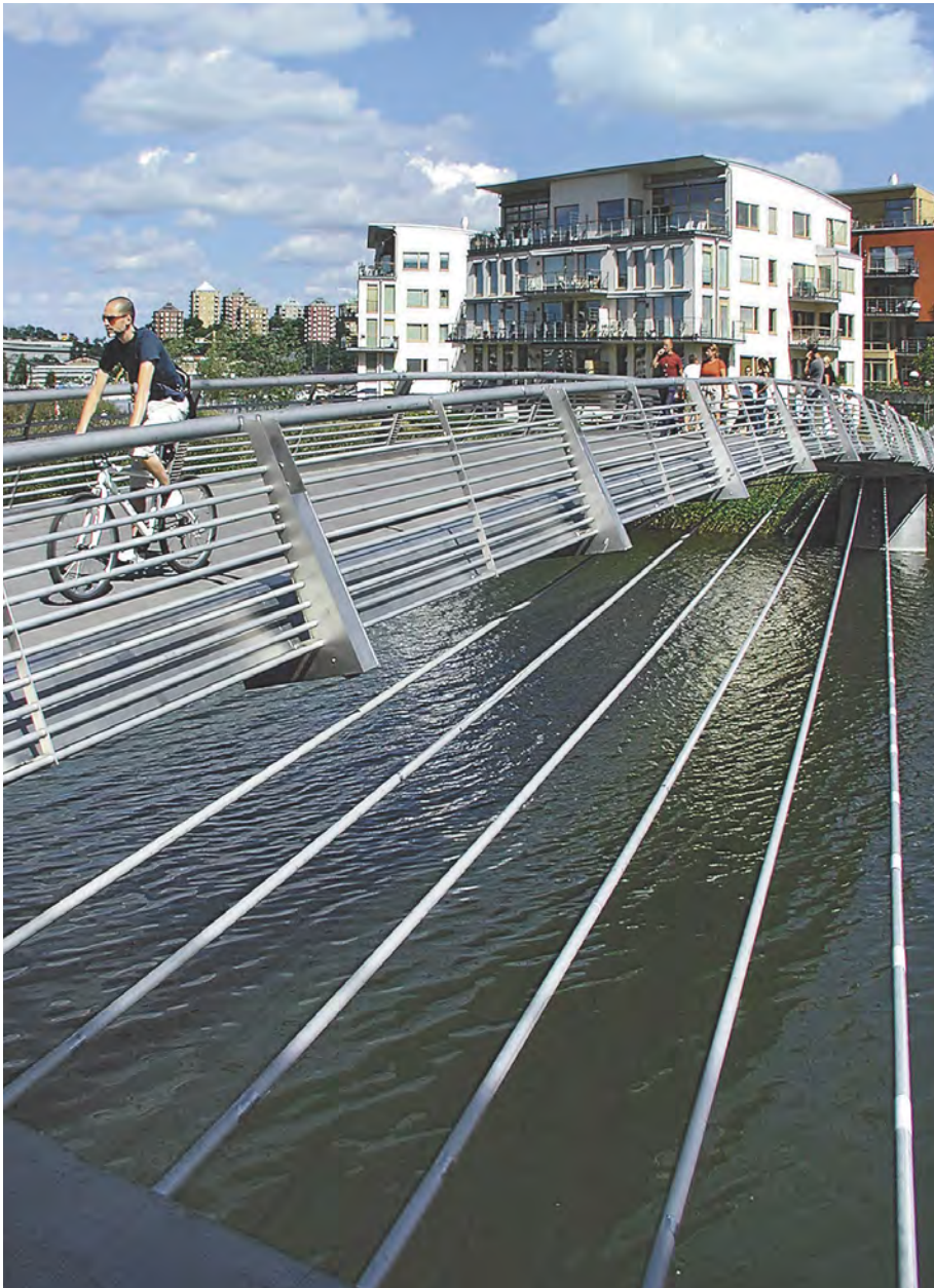
Duplex stainless steel bridge in Stockholm, Sweden. © Outokumpu
