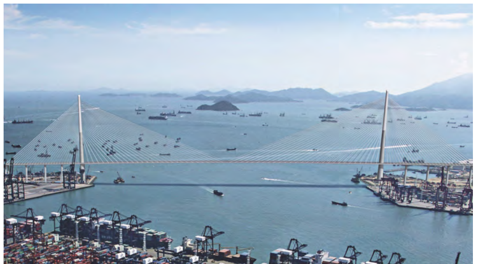
Stonecutters Bridge, Hong Kong. © Ove Arup & Partners
