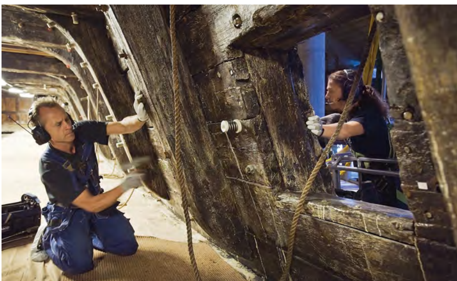
Installation of hyper duplex stainless steel bolts to preserve the historic wooden Vasa ship in Sweden. © Anneli Karlsson, the Swedish National Maritime Museums
