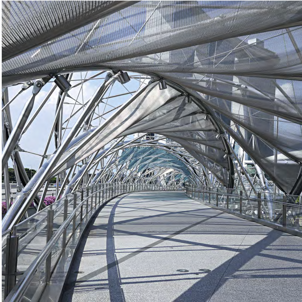
The Helix Bridge, Singapore, made of 2205 duplex stainless steel.
