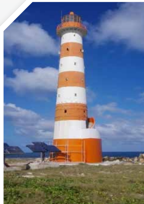
Morant Point Light Tower powered by Solar Panel and Wind Turbine
