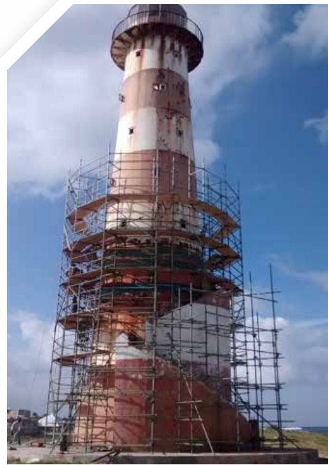
Morant Point Light Tower under renovation
