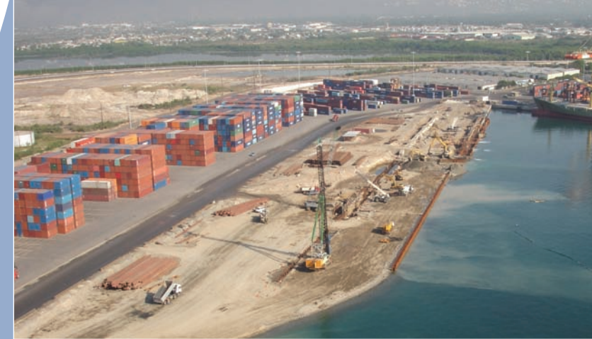
Work progresses apace on the new Western Berth at the KCT.
