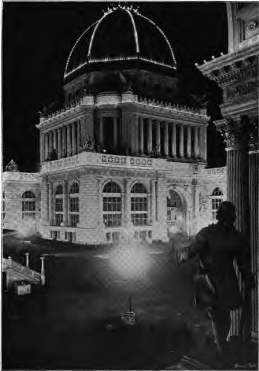
ADMINISTRATION BUILDING.—LOOKING FROM ELECTRICITY BUILDING.
