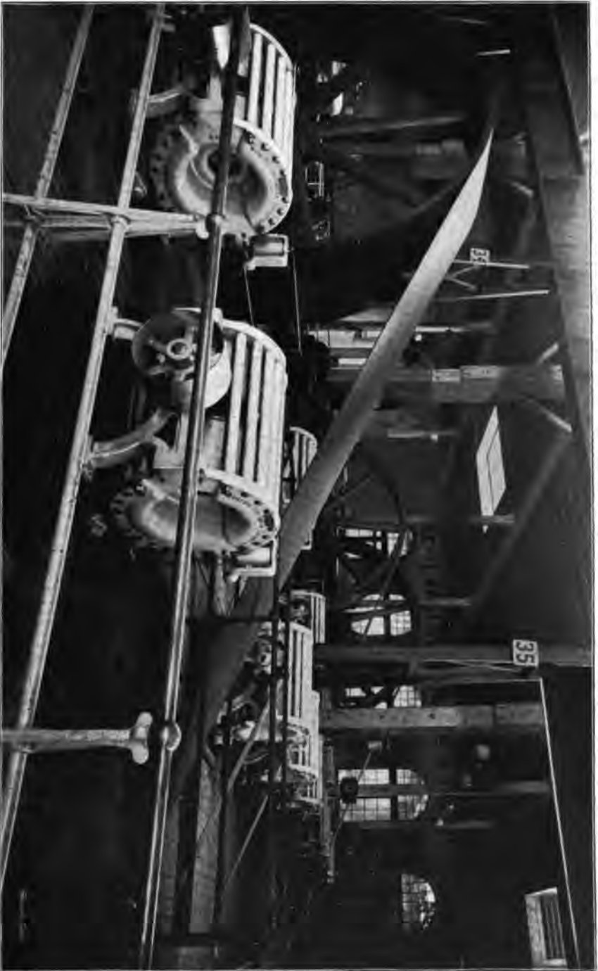
THOMSON-HOUSTON POWER PLANT.—MACHINERY HALL.
