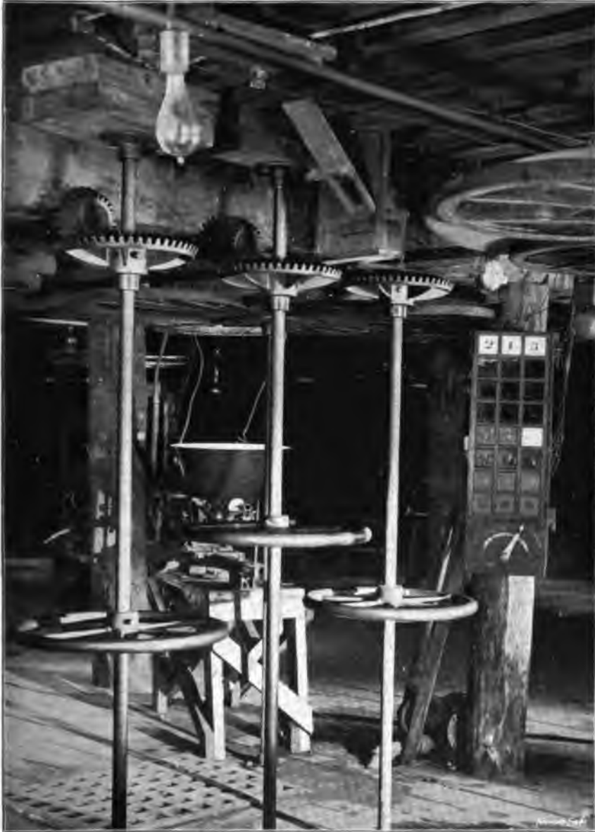
INTERIOR VIEW OF ELECTRIC FOUNTAIN.—SIGNAL SLIDES.
