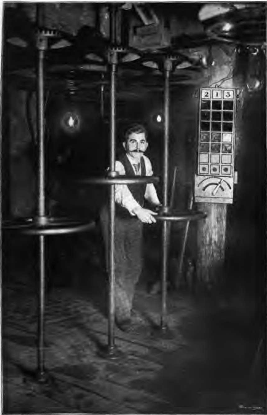
INTERIOR VIEW OF ELECTRIC FOUNTAIN.—CHANGING THE COLORS.
