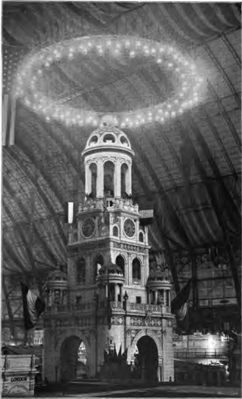
GREAT CORONA.—CENTRE MANUFACTURES BUILDING.
