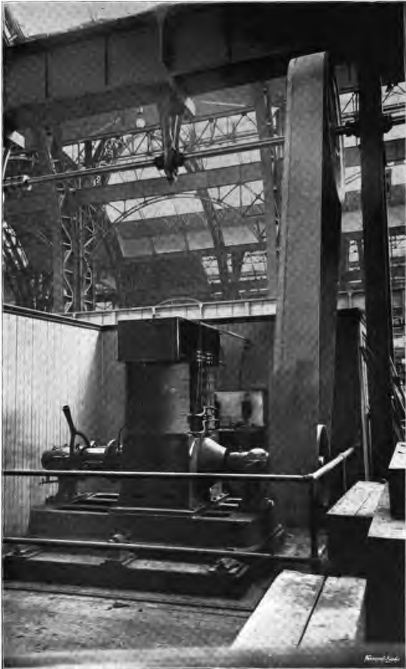
115 H.-P. EDISON MOTOR DRIVING LINE SHAFTING. MACHINERY HALL.
